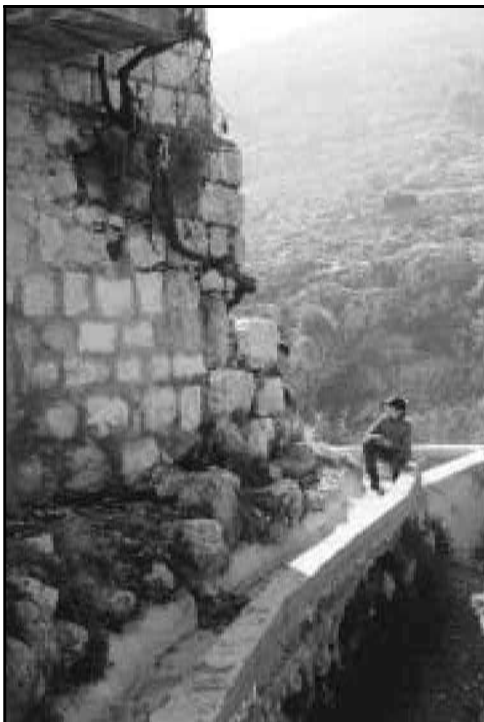
New irrigation channel on top of 8in sewage pipe passing the PHG project office in Artas
