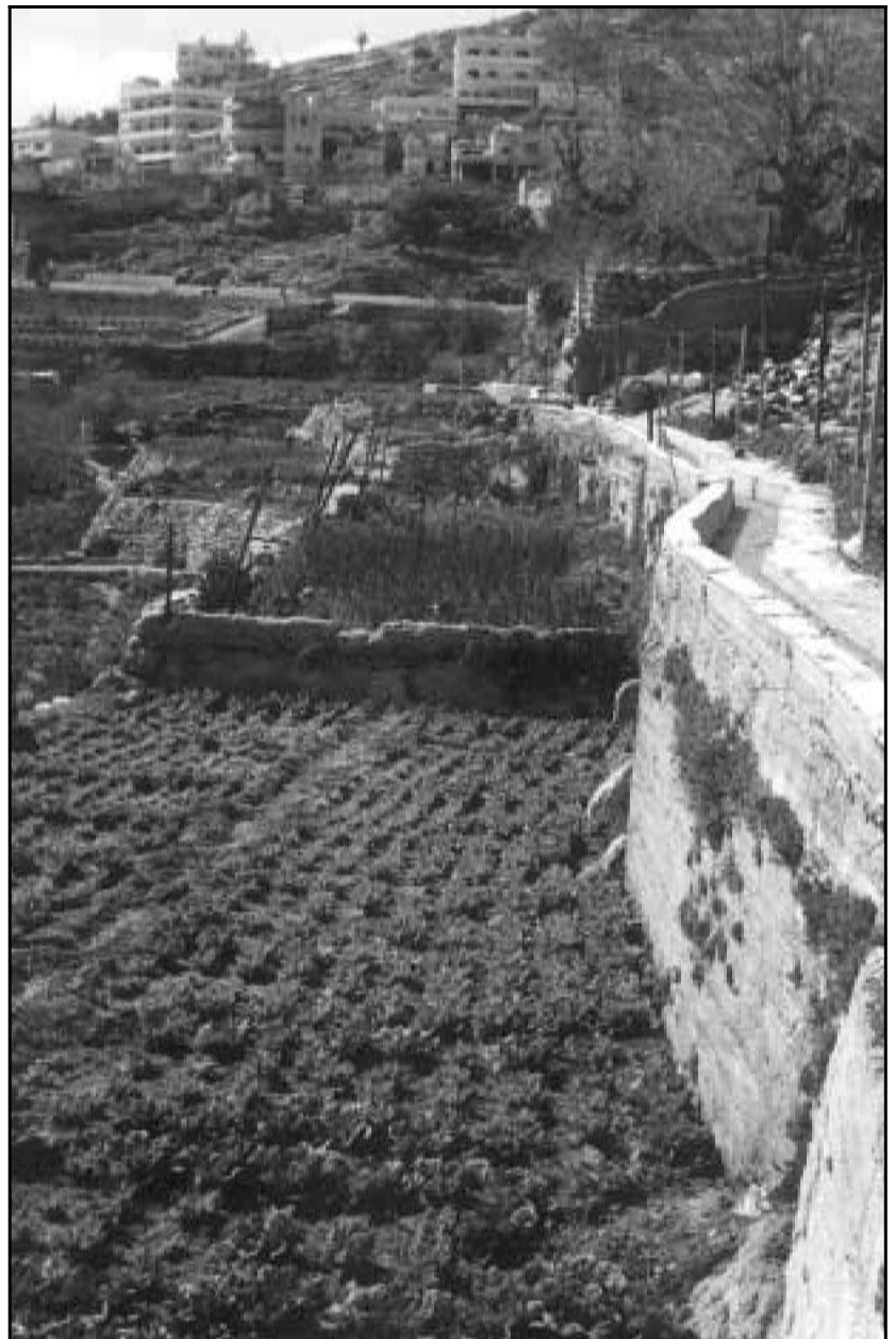
New irrigation channel on top of 8in sewage pipe passing village lettuce beds
