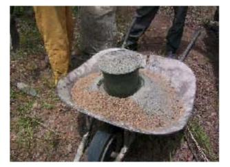
The sand and cement must be very well mixed. After mixing the dry sand and cement add water(about 2 - 3 litres) to make a stiff mix.
