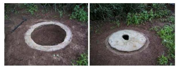
Dig down hole within the ring beam to at least 1 metre below surface. Place soil around ring beam and ram in place hard. Add leaves to pit base. Lay anthill mortar or weak cement on ring beam and place slab on top. Bed in and level the slab. The structure can now be built around the slab.
