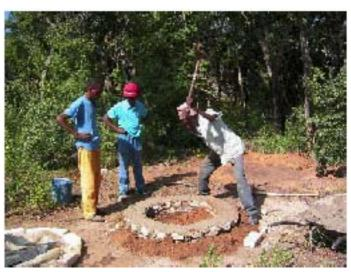
This ring beam and soil helps to raise the toilet above ground level and stops rain getting into the pit. The ring beam and surrounding soil helps to make the toilet stronger.
