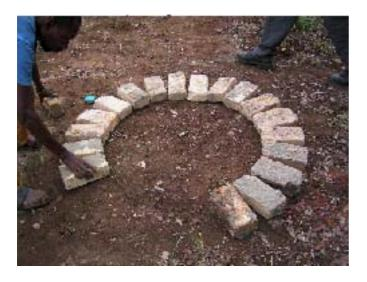
Now make up some ant hill mortar (Ivhu re pa churi) by breaking up ant hill soil and mixing with water. Using a trowel add the anthill mortar between and above the bricks.
