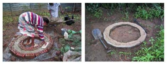
Add remainder of concrete mix, level off and ram flat with wooden float. Cover with plastic sheet and leave to cure for 10 days. Keep wet at all times. Then move to location on level ground.
