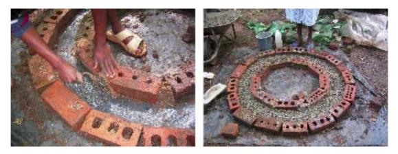
Fill in spaces between inner circle of brick mould with wet sand. Make the 6:1 mix of clean river sand and fresh cement. Add half the mix, level off and then add the circle of 3 – 4mm wire.
