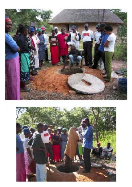
First put a big sack full of dry leaves in the pit. The leaves will help the contents of the pit to compost. Then lay the slab over the ring beam. It is best to lay the slab in some mortar placed on the ring beam. This can be made of anthill mortar or weak cement and sands (20:1).
