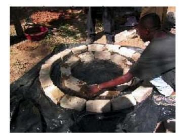
Once the brick mould has been made, make up the concrete mixture of 5 litres fresh cement with 30 litres good river sand. Mix the dry parts thoroughly first then mix with about 3 litres fresh water. Mix thoroughly again. Add half of this mixture to the mould. Then take a length of 3 - 4mm wire and place above the concrete mix about half way between the inner and outer bricks.
