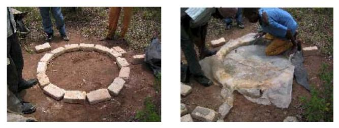
A sheet of plastic is laid in the mould
