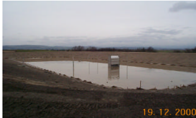
Figure 2.7. The first lagoon during construction
