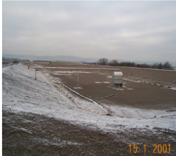
Figure 2.9. The second lagoon during construction
