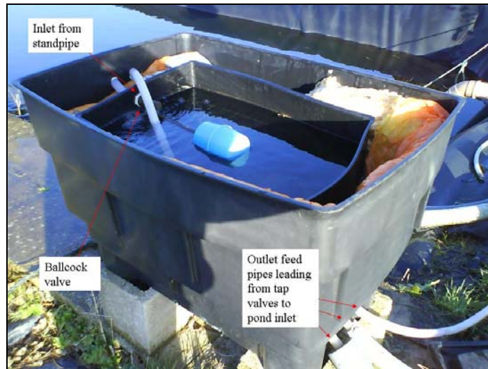
Figure 4.2: The cold water storage tank used to control the flow of fresh water into the PFP's.
