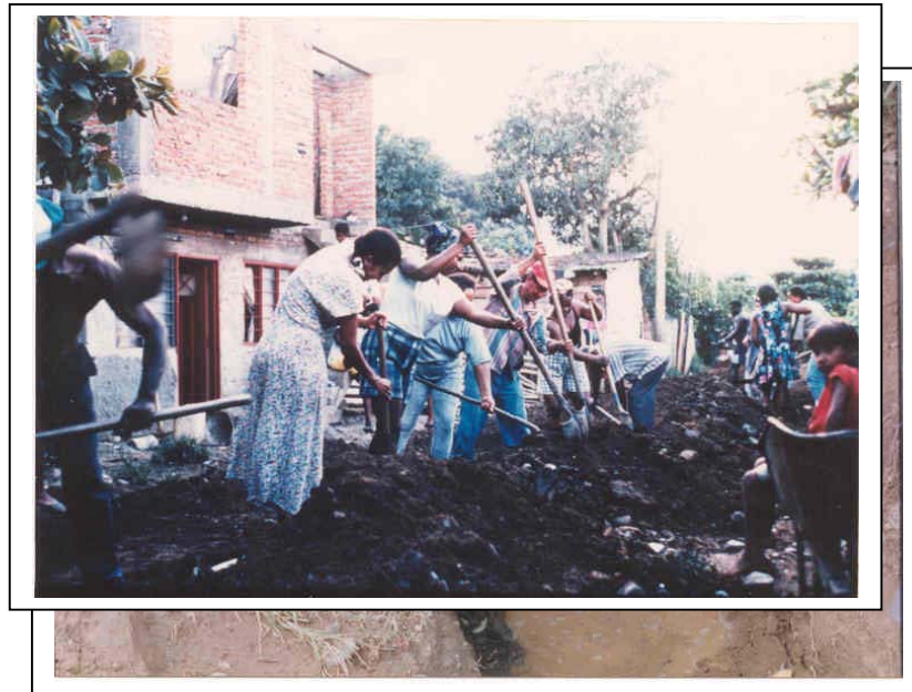
Photograph 26 Part of the water network was cleaned
