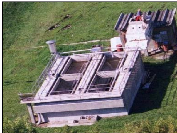
Figure 3.5 Aerial view of the UASB reactor at the Ginebra research station.
