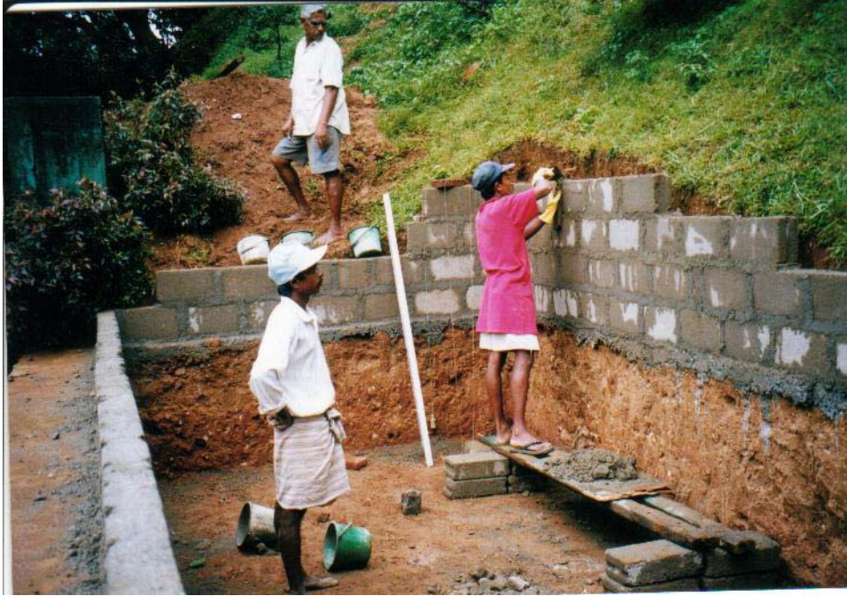
Plate 5-5. A retaining wall being built to protect a VFPGF unit.
