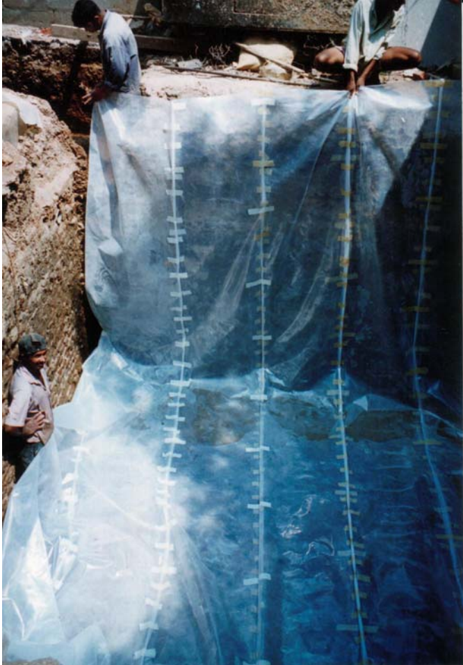
Plate 5-4. The assembled liner being placed in the excavation for the bed
