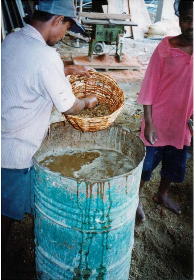
Plate 5-3. Bed media being washed by immersion in water.
