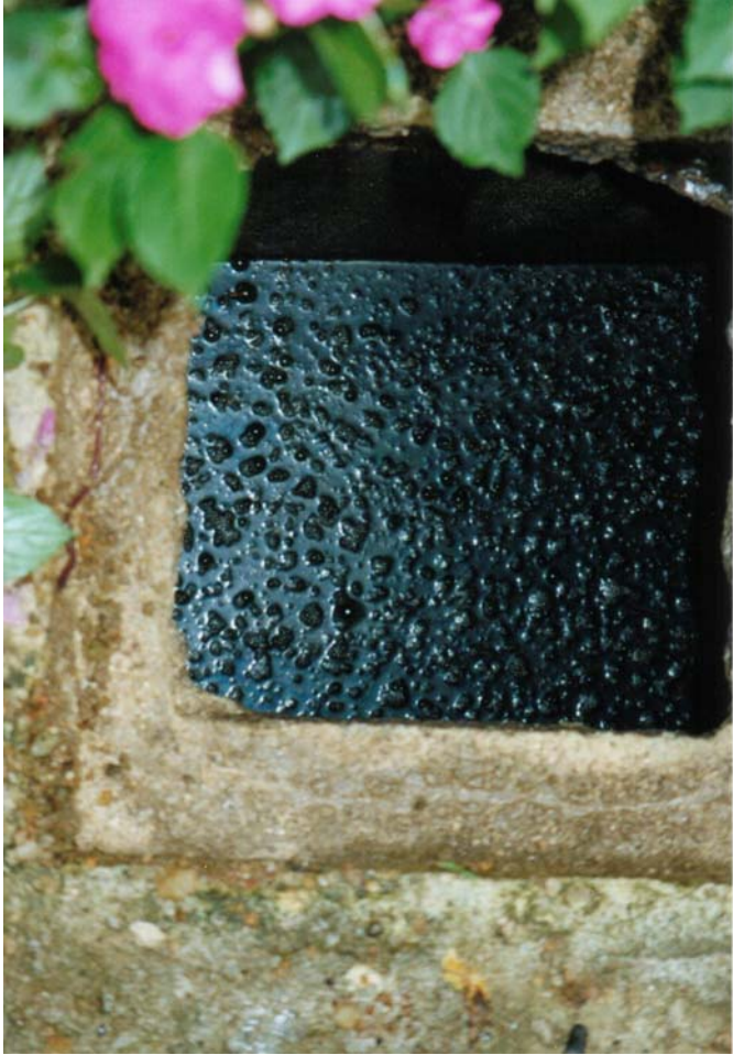
Plate 5-6. Visible bubbling of the water surface in an anaerobic filter
