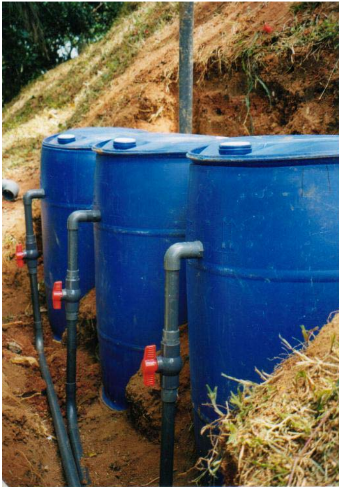
Plate 5-2. Dosing siphons fabricated with plastic barrels
