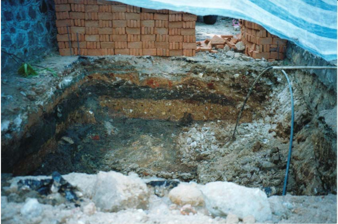
Plate 4-11. The excavation for the percolation bed intersecting the black soil layer.
