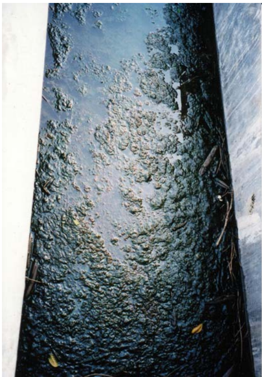
Plate 4-6. A completely clogged reed bed channel.
