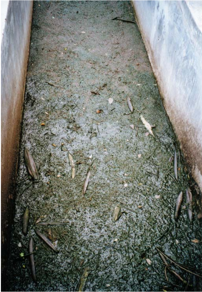
Plate 4-7. The biomat layer soon after releasing the stagnant water.
