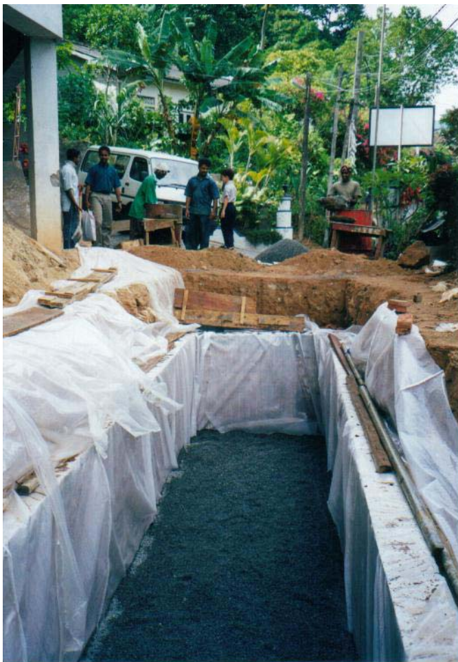
Plate 4-3. The percolation bed being re-laid with stone chips.
