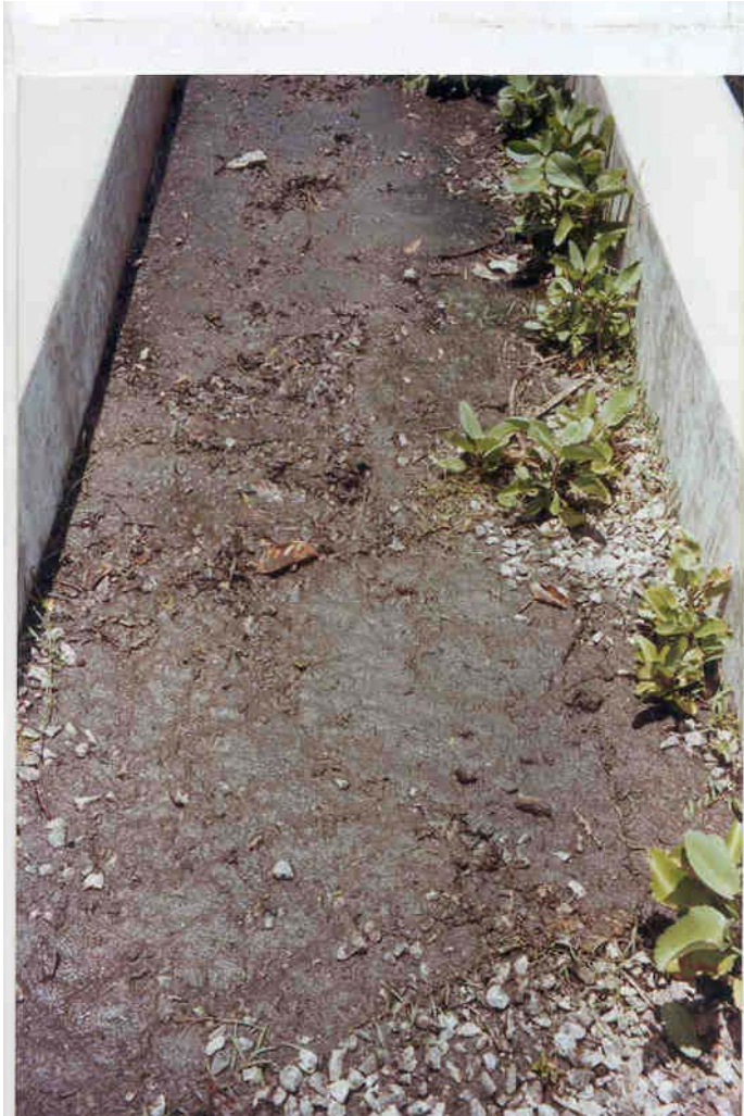
Plate 4-16. A view of the channel immediately after clearing the clogged area
