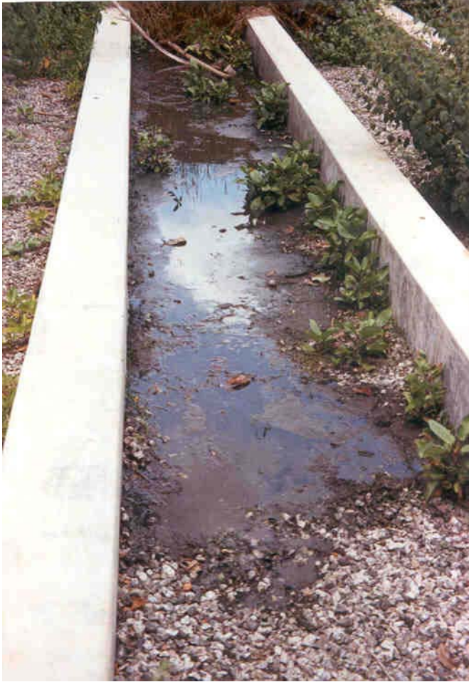
Plate 4-15. A close up view of the clogged area of the reed bed.
