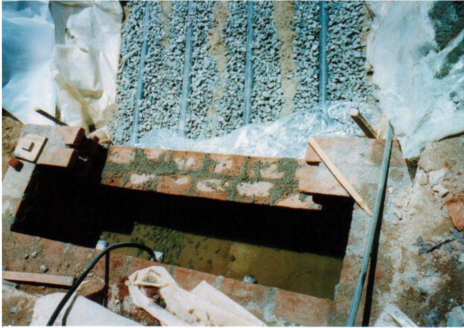
Plate 4-2. The new arrangement of the effluent collector pipes being laid.
