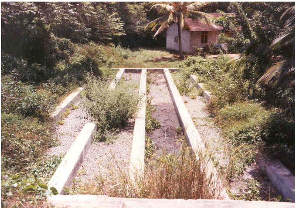
Plate 4-14. The Ranpokunugama reed beds after eight months of operation
