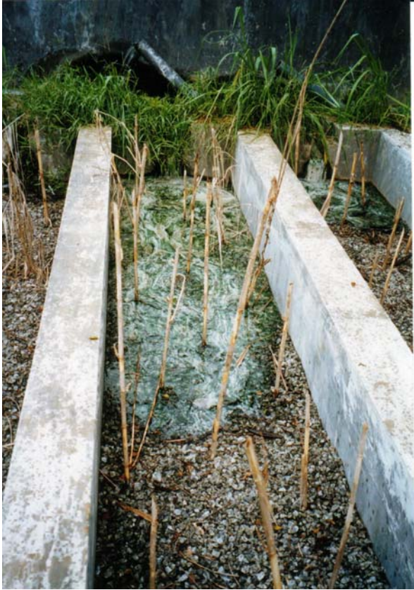
Plate 4-8. The reed stems a couple of days after planting
