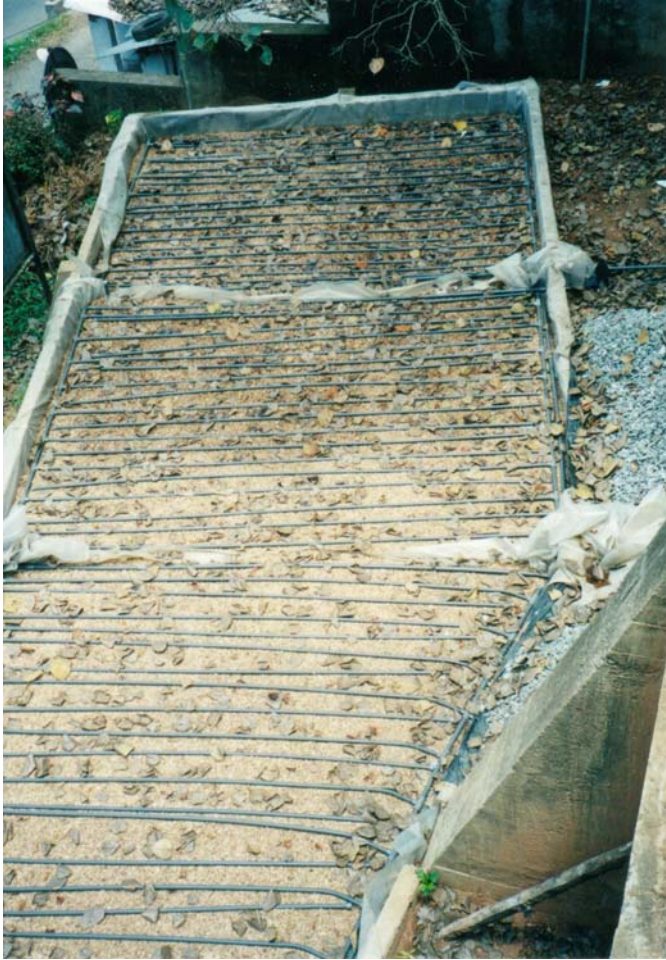
Plate 3-13. A view of the same area with the VFPGF unit in place, prior to planting.
