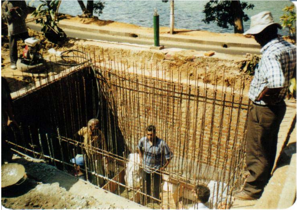
Plate 3-9. The anaerobic filter unit during construction.
