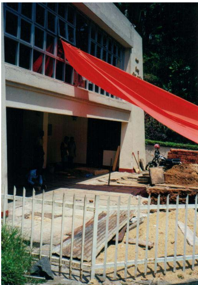
Plate 3-53. The anaerobic filter under construction at Sampath Hall.
