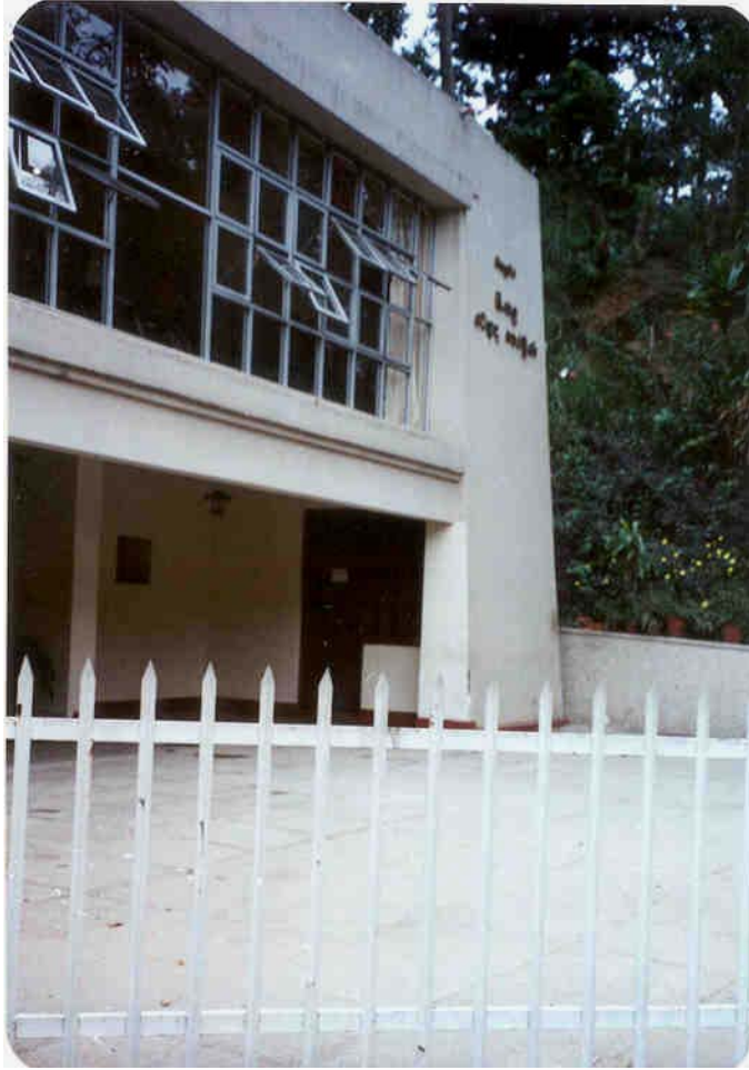
Plate 3-54. The entrance forecourt after completion of construction
