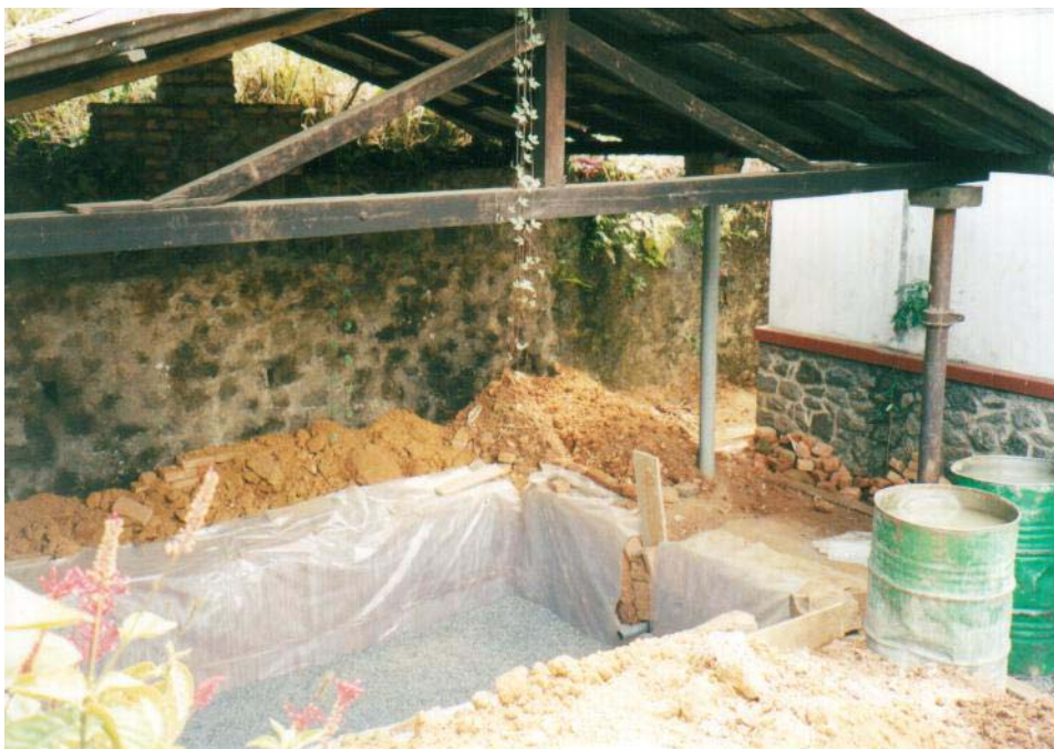
Plate 3-24. The percolation bed being laid under the garage floor.
