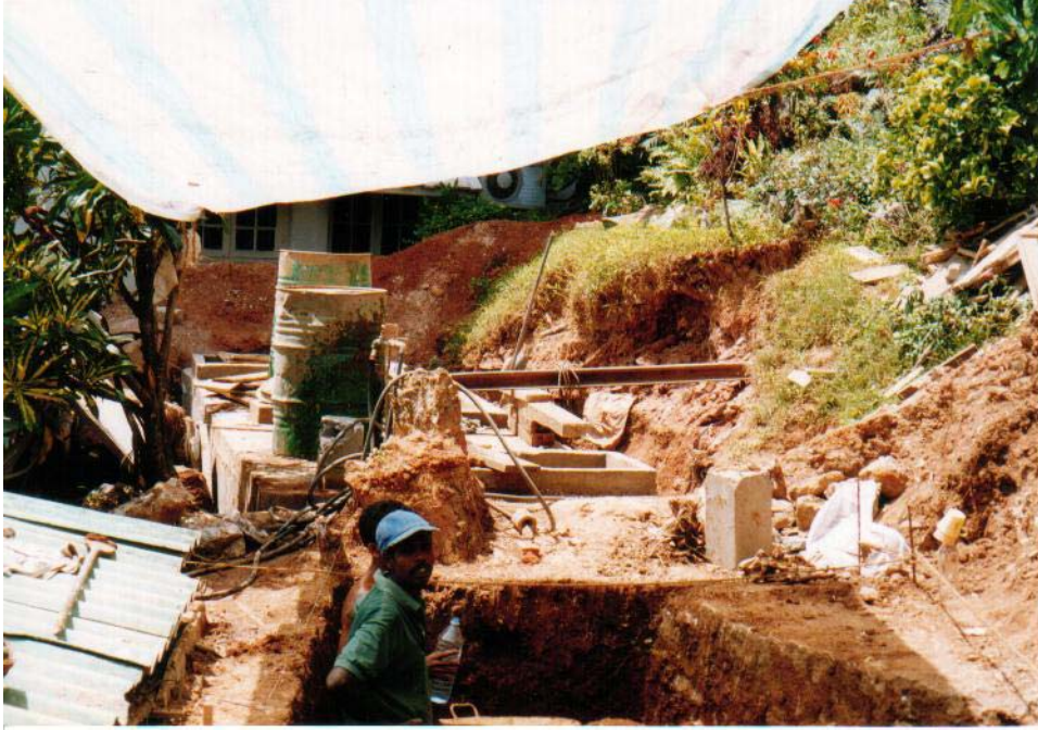
Plate 3-35. The treatment units under construction.
