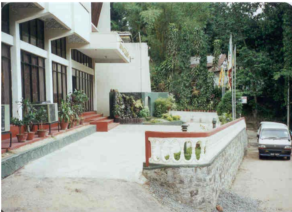
Plate 3-10. A view of the driveway after construction was completed.
