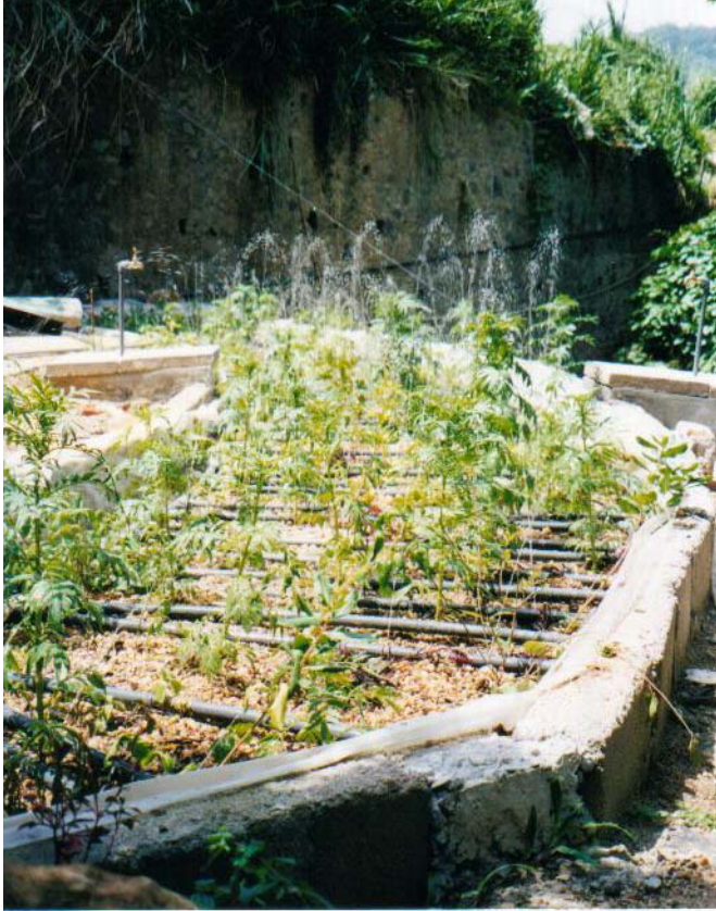
Plate 3-20. Influent dosing in progress soon after commissioning.
