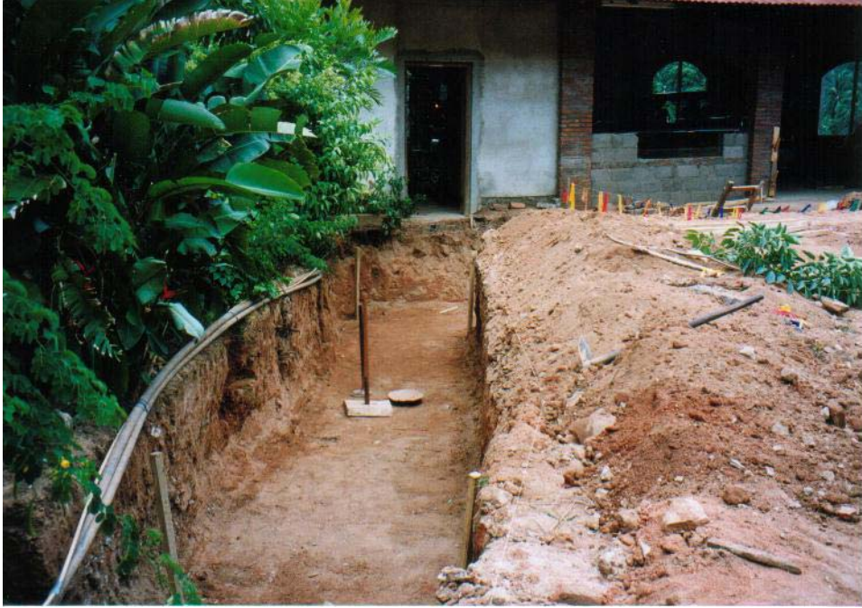
Plate 3-3. Excavation for the VFPGF unit for system 2 during construction stage.
