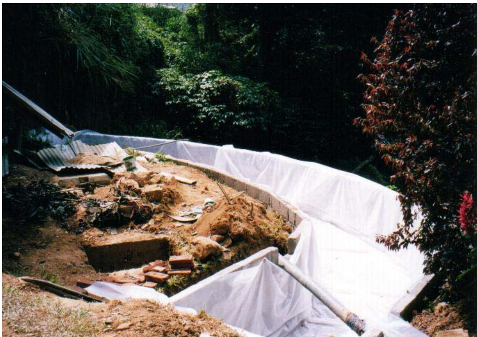
Plate 3-19. The VFPGF unit of System 2 under construction.
