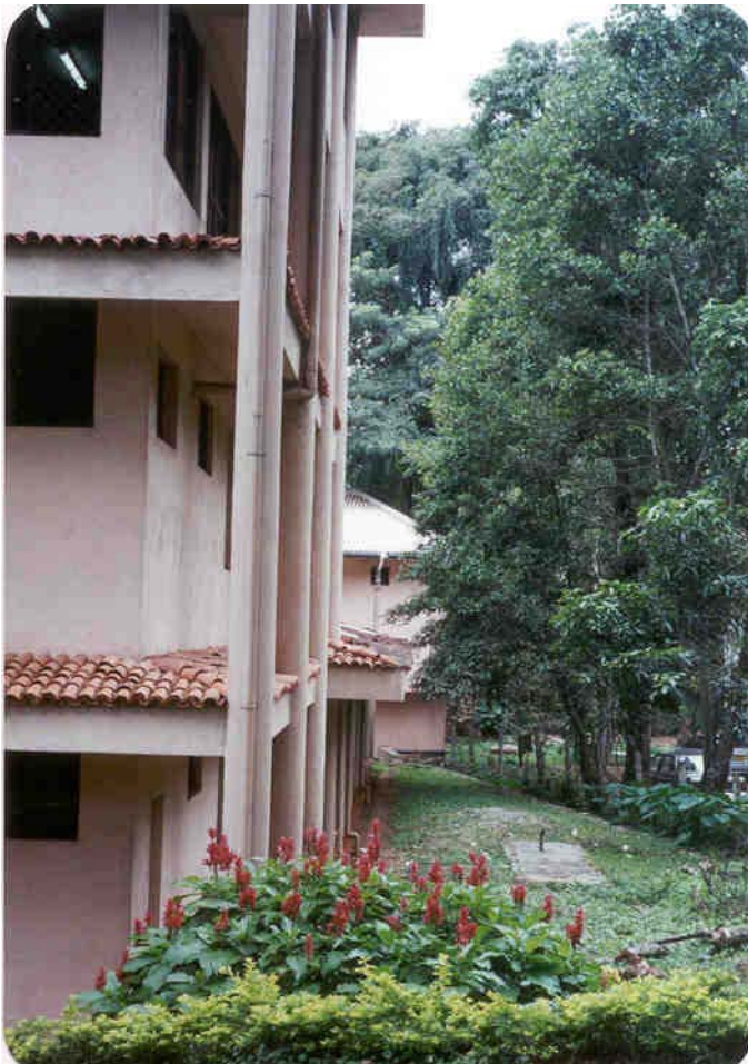
Plate 3-56. A view of the PGIA Library complex with the anaerobic filter beside it.
