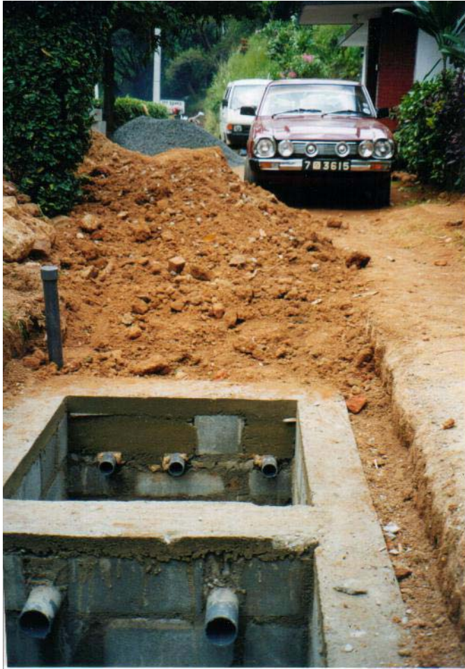
Plate 3-23. The combined septic tank-anaerobic filter unit during construction
