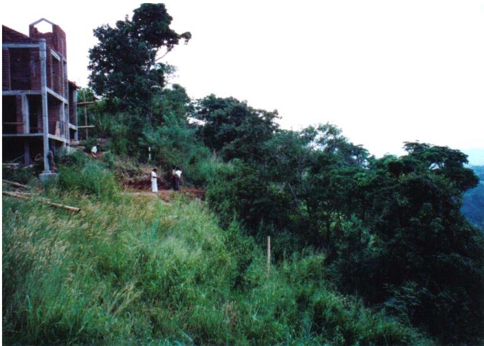
Plate 3-36. Site for treatment units prior to commencement of construction
