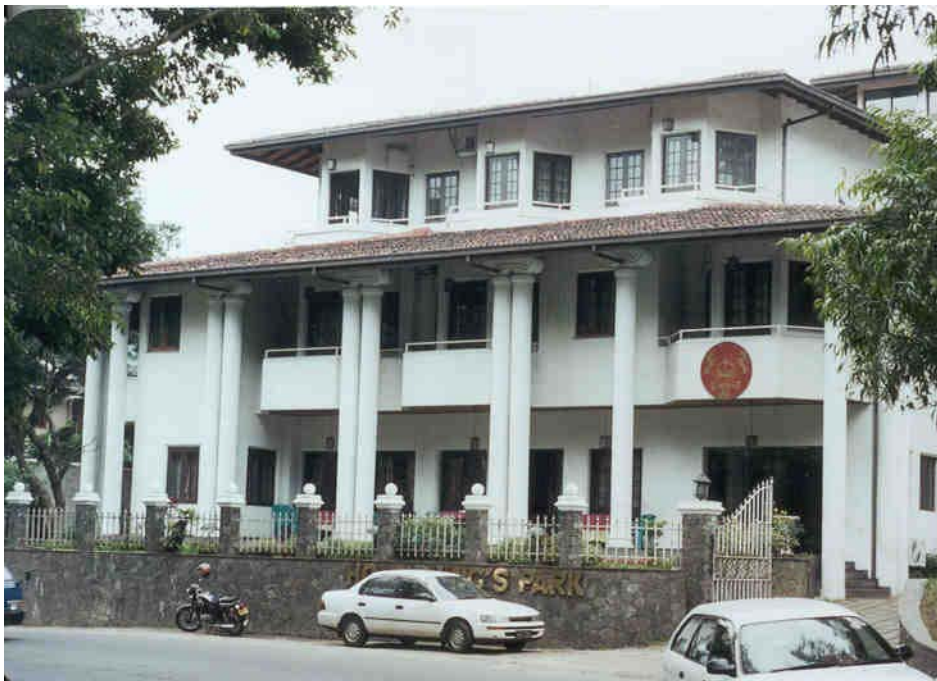
Plate 3-25. A view of the hotel building
