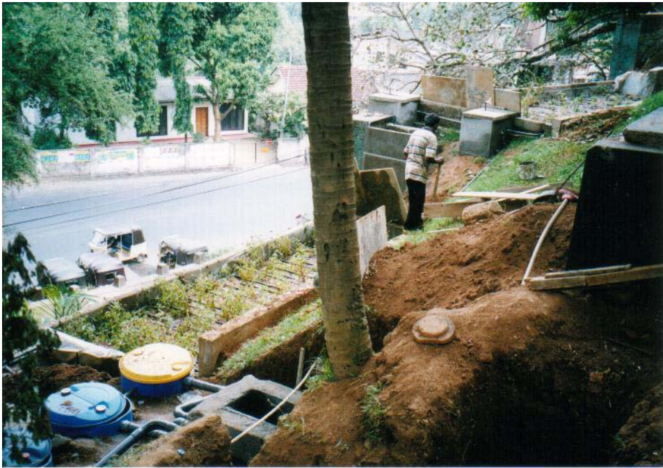
Plate 3-15. The second VFPGF during construction.
