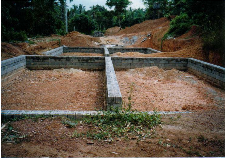
Plate 3-43. One of the reed bed systems during early stages of construction.
