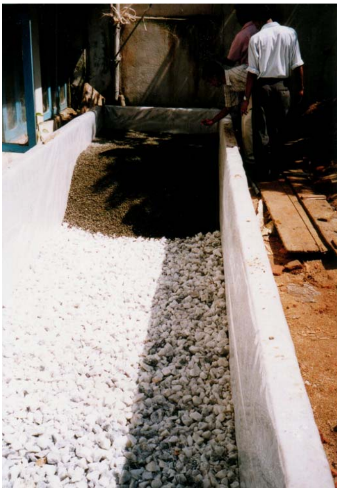
Plate 3-32. The VFPGF unit with the bed partially laid.
