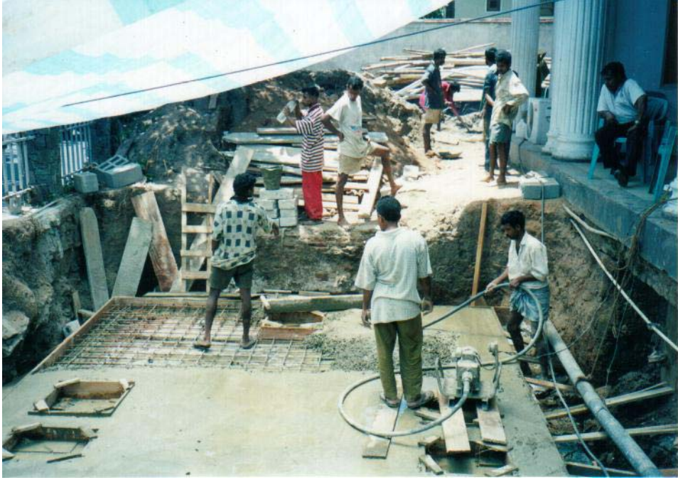
Plate 3-26. The cover slab of the anaerobic filter being laid during construction
