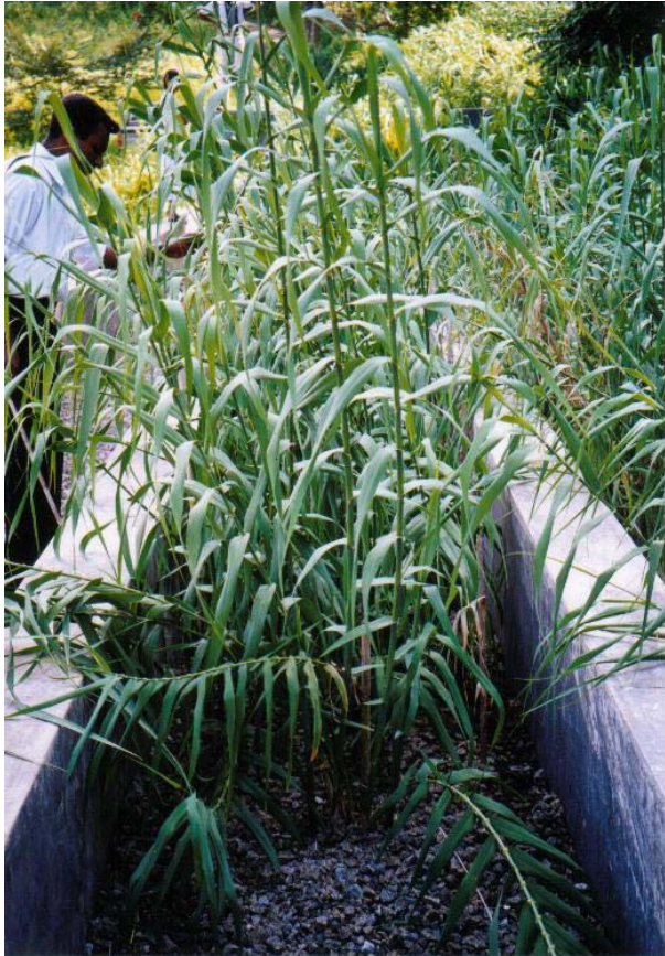
Plate 3-49. A vegetated reed bed channel at Akbar-Nell.
