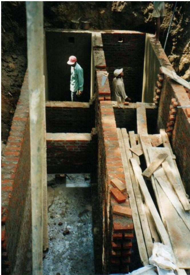
Plate 3-51. The combined septic tank-anaerobic filter under construction.
