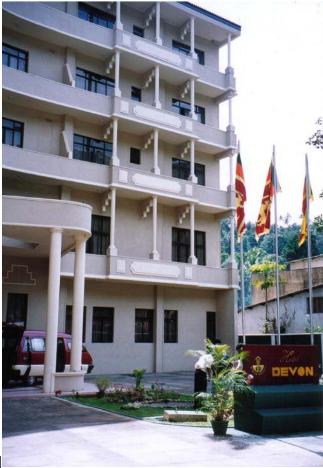
Plate 3-6. A view of the hotel building.
