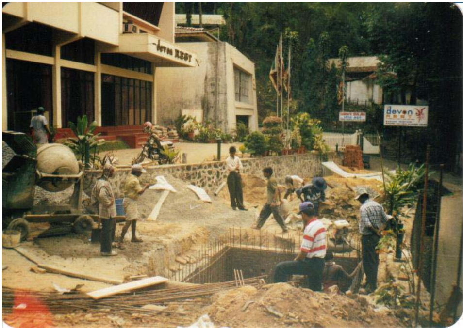
Plate 3-8. Hotel entrance and driveway during construction of the anaerobic filter unit.
