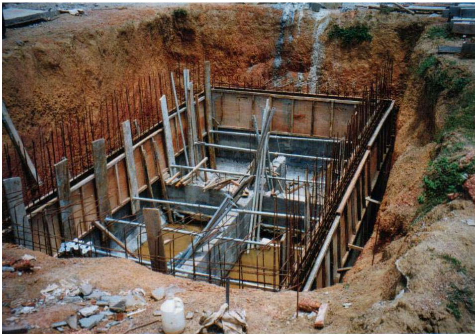
Plate 3-42. A septic tank unit under construction
