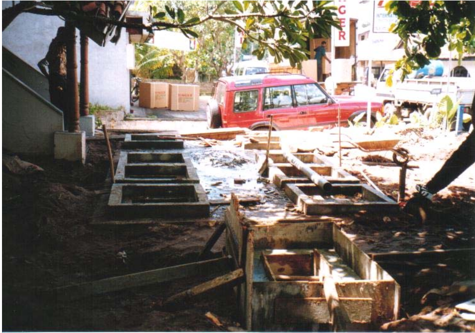
Plate 3-31. Combined septic tank-anaerobic filter unit nearing the end of construction
