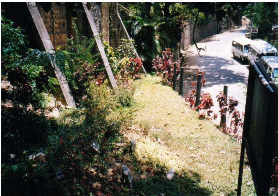
Plate 3-12. Area where the lower VFPGF unit was located prior to construction.
