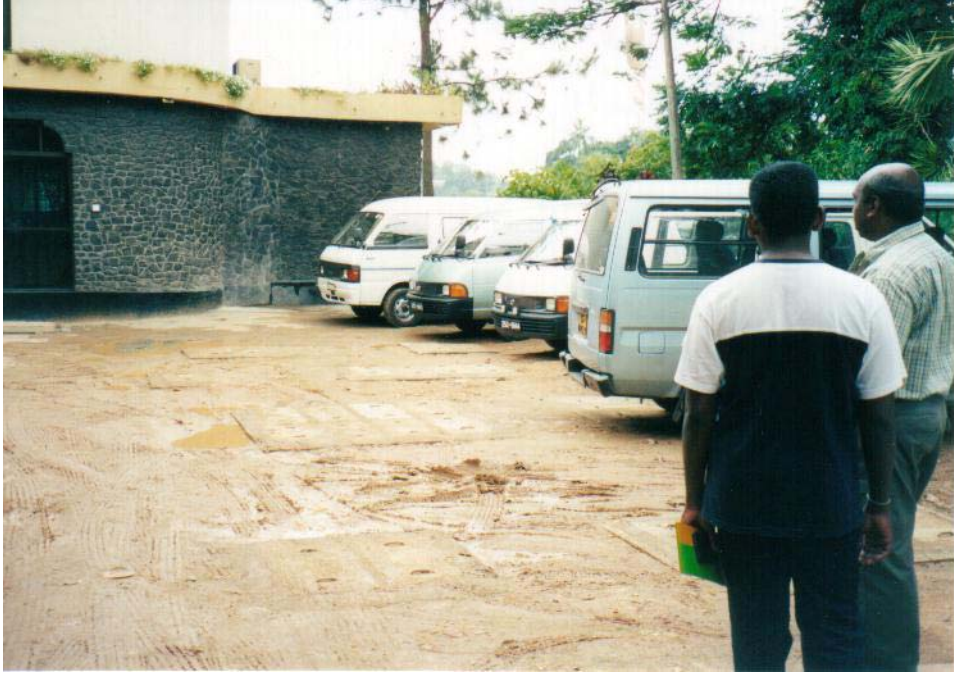
Plate 3-17. The same parking area soon after construction of the septic tank – anaerobic filter unit.
