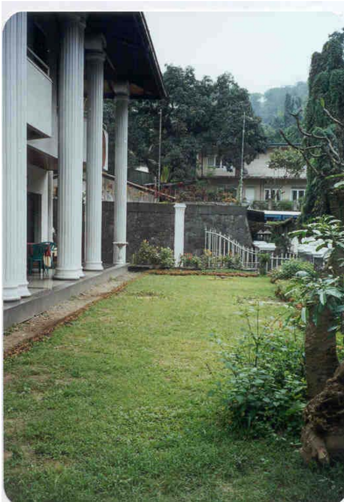
Plate 3-27. The same area after construction and relaying of the lawn.
