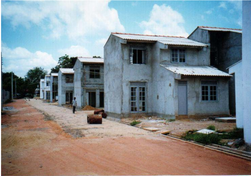
Plate 3-41. Luisawatte housing scheme under construction
