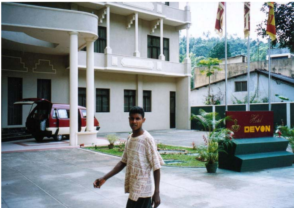
Plate 3-5. View of the hotel forecourt area under which the treatment units are located
