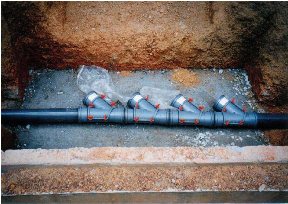
Plate 3-45. House connections with removable cleaning doors during installation.
