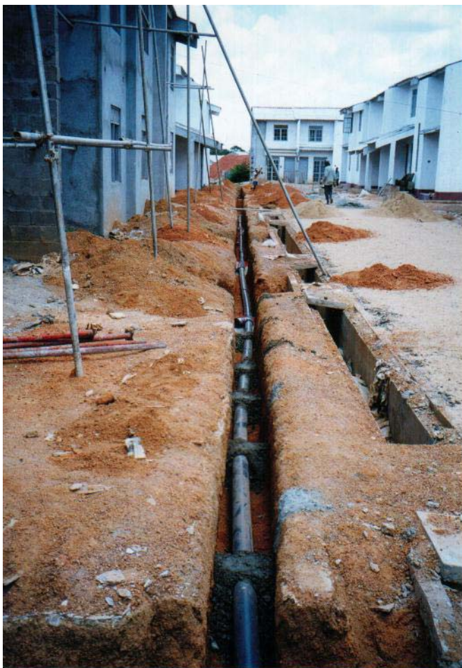
Plate 3-44. A simplified sewer line being laid.
