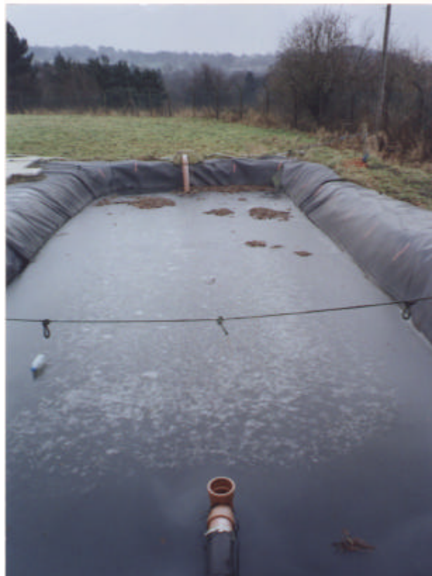
Figure 5.50 Leaves accumulating around the inlet of the Red pond (winter 2001)
