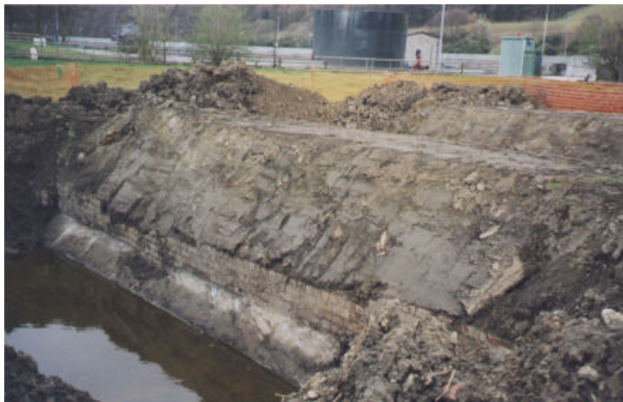
Figure 4.2 Formation of the ponds and embankments
