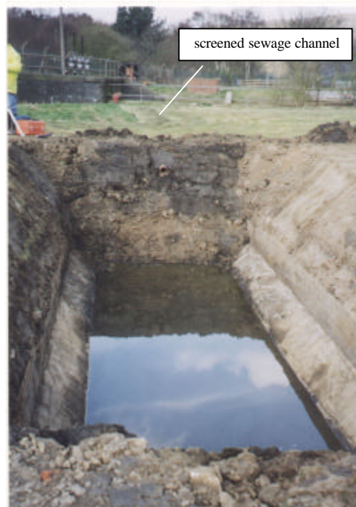
Figure 4.1 An excavation before lining
