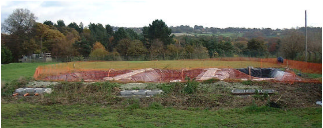
Figure 4.7 The pilot-scale facultative ponds after completion
