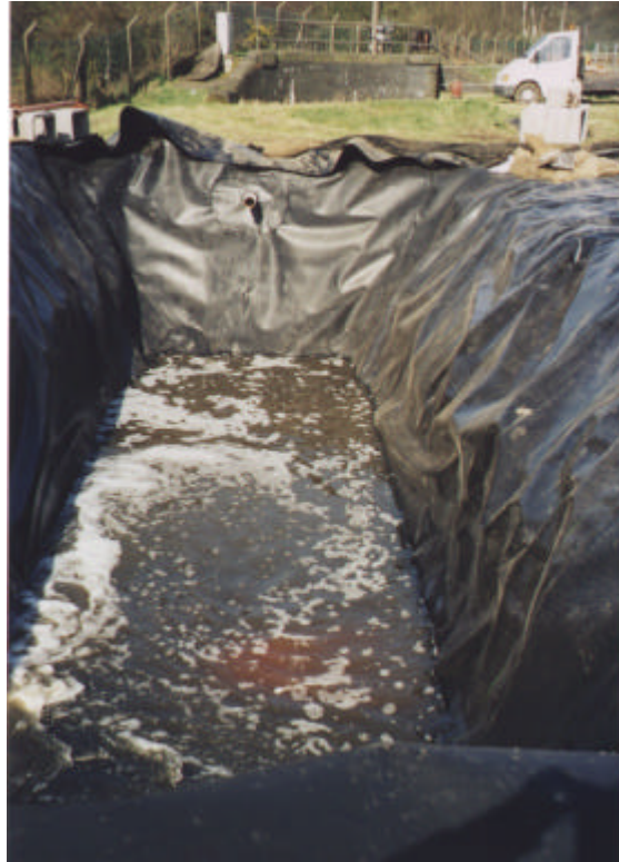
Figure 4.3 An excavation with the HDPE liner fitted
