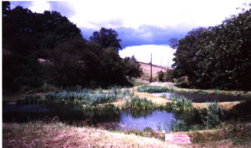
Figure 3.7 Ponds 2 and 3 at the Botton Village System
