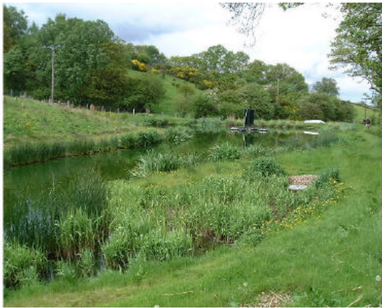
Figure 3.3 The facultative pond at Botton Village, North Yorkshire
