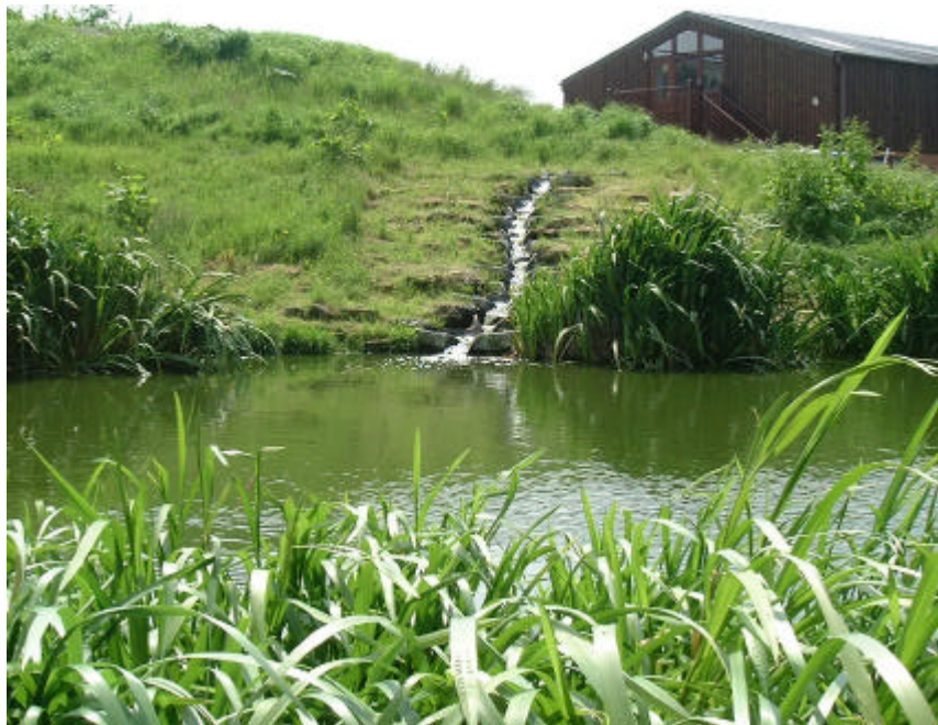
Figure 3.9 The facultative pond at the Larchfield (Wheelhouse) system
