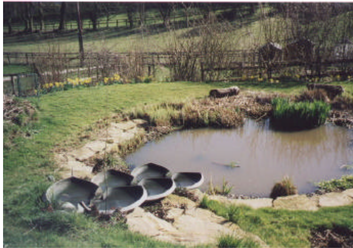
Figure 3.2 The flowform cascade to the facultative pond at Spring Cottage, Wiltshire.
