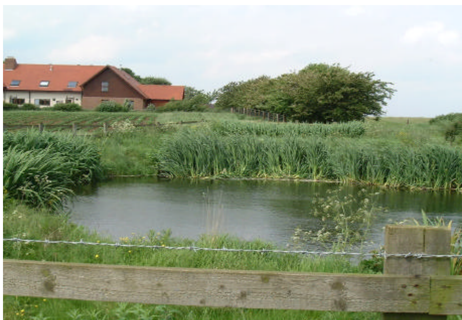
Figure 3.10 The facultative pond at the Larchfield (Levenhouse) system
