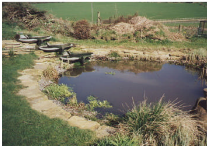
Figure 3.6 The facultative pond at Spring Cottage.
