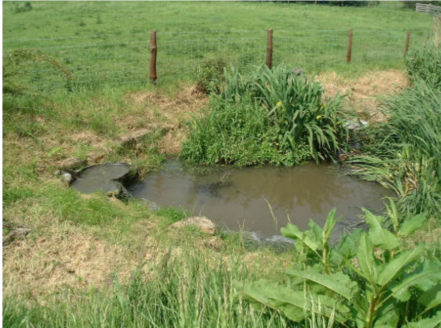
Figure 3.8 The anaerobic pond at the Larchfield (Wheelhouse) system
