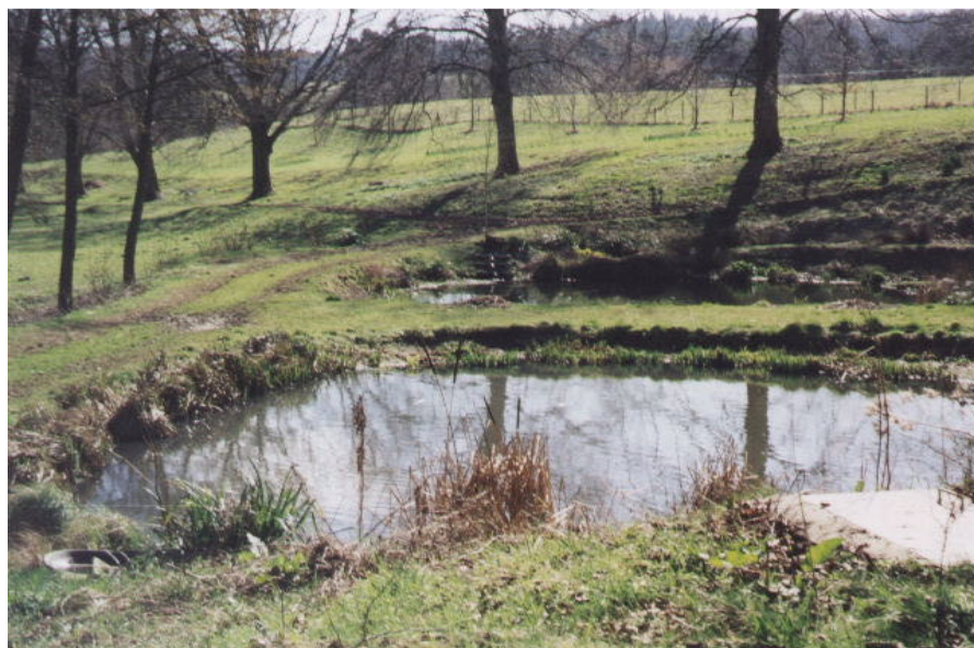
Figure 3.5 The system at Halewell Hotel with the facultative pond in the foreground
