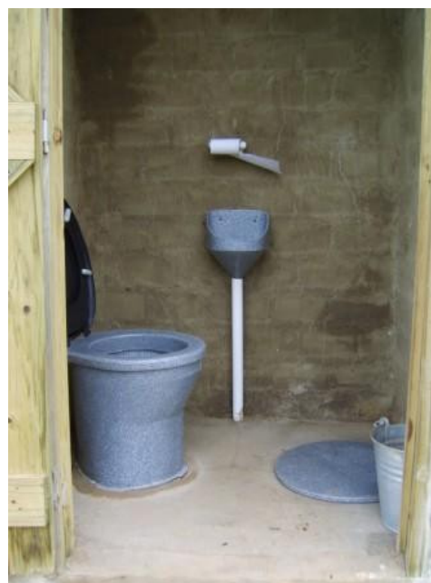
Figure 2. Front view of eThekwini UD-VIV latrine with the door open, showing the UD-pedestal seat and urinal, also the closed-off entrance to the vault not in use
