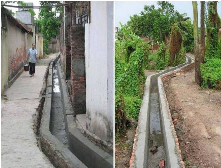
Low-cost combined drainage at Lai Xá, Vietnam
