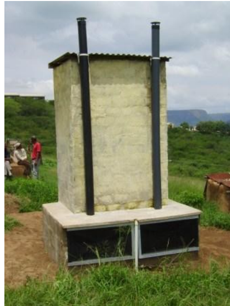
Figure 4. Rear view of eThekweni UD-VIV latrine, showing the two above-ground separately ventilated vaults and, between them, the pipe taking the diverted urine to an adjacent soakaway.
