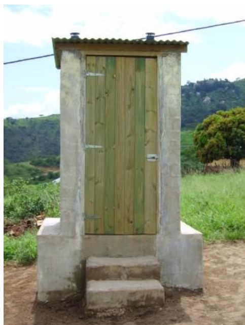
Figure 1. Front view of eThekwini UD-VIV latrine.
