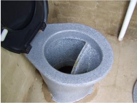
Figure 3. Close-up view of the UD-pedestal seat (front compartment for urine, rear compartment for faeces).
