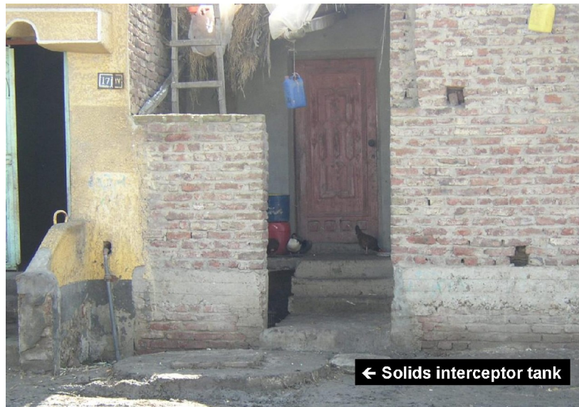
Figure 2. A village house in the Nile Delta, Egypt with its solids interceptor tank.
