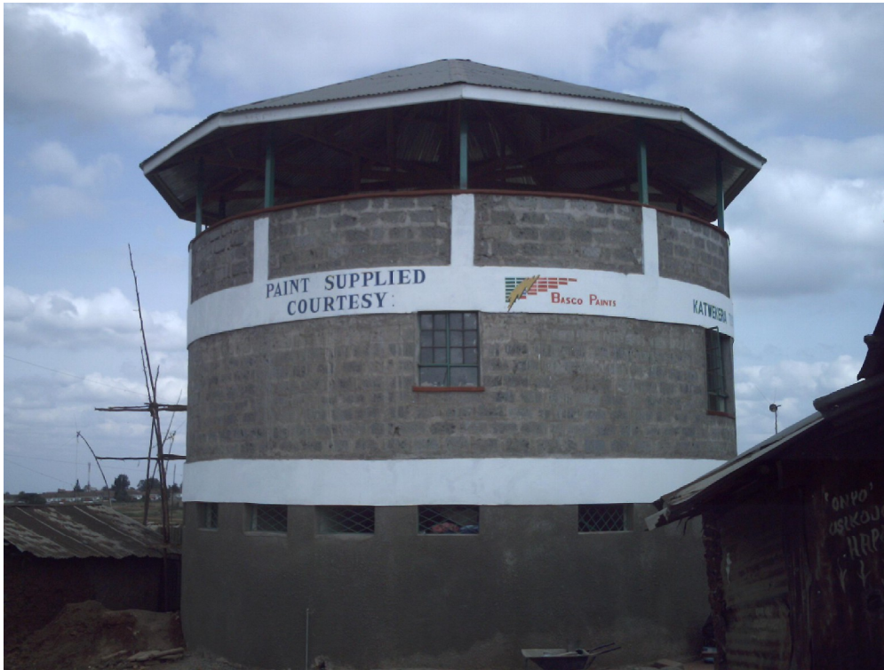
Figure 1. Community-managed sanitation block in Gatwekera village, Kibera, Nairobi. The ground floor is the sanitation compartment, and the top floor is a 'community room' used for meetings, weddings, parties, etc. Underneath the ground floor is ...
