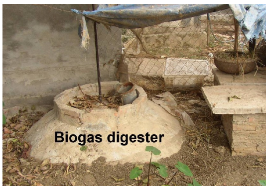
3. Household anaerobic digester for biogas generation and collection
