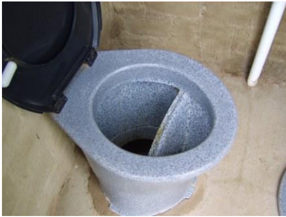
Figure 3. Close-up view of the UD-pedestal seat (front compartment for urine, rear compartment for faeces).
