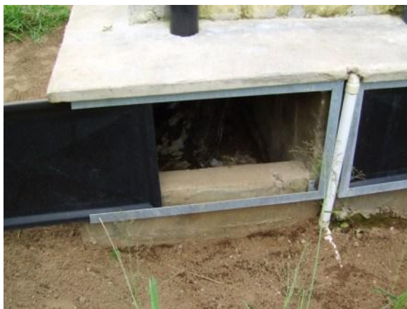
Figure 5. Close-up of one of the vaults with its sliding door partially open. The urine-diversion pipe is clearly visible on the right.
