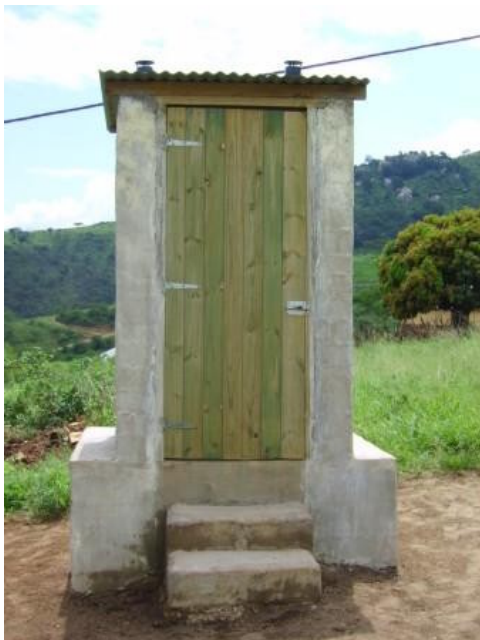
Figure 1. Front view of eThekwini UD-VIV latrine.
