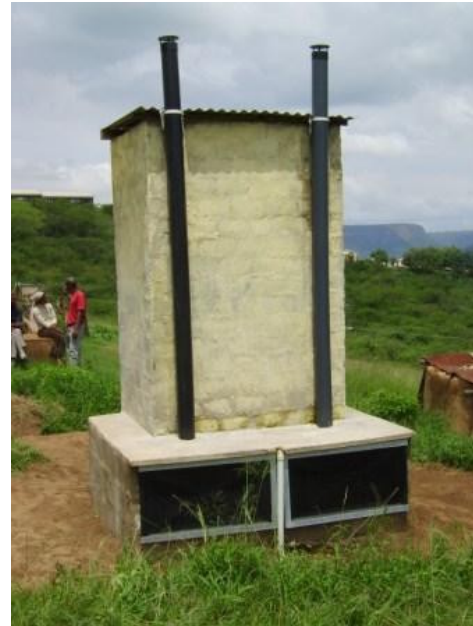
Figure 4. Rear view of eThekweni UD-VIV latrine, showing the two above-ground separately ventilated vaults and, between them, the pipe taking the diverted urine to an adjacent soakaway.
