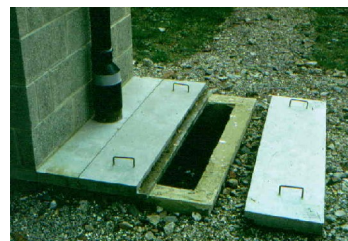
Figure 2. An alternating twin-pit VIP latrine. Each of the two pits has its own 100-mm diameter vent pipe with a fly screen at its top. The external pit cover slabs are only weakly mortared so they can be easily removed when the pit is to be emptied:
