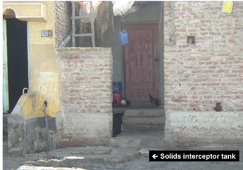
Figure 2. A village house in the Nile Delta, Egypt with its solids interceptor tank.
