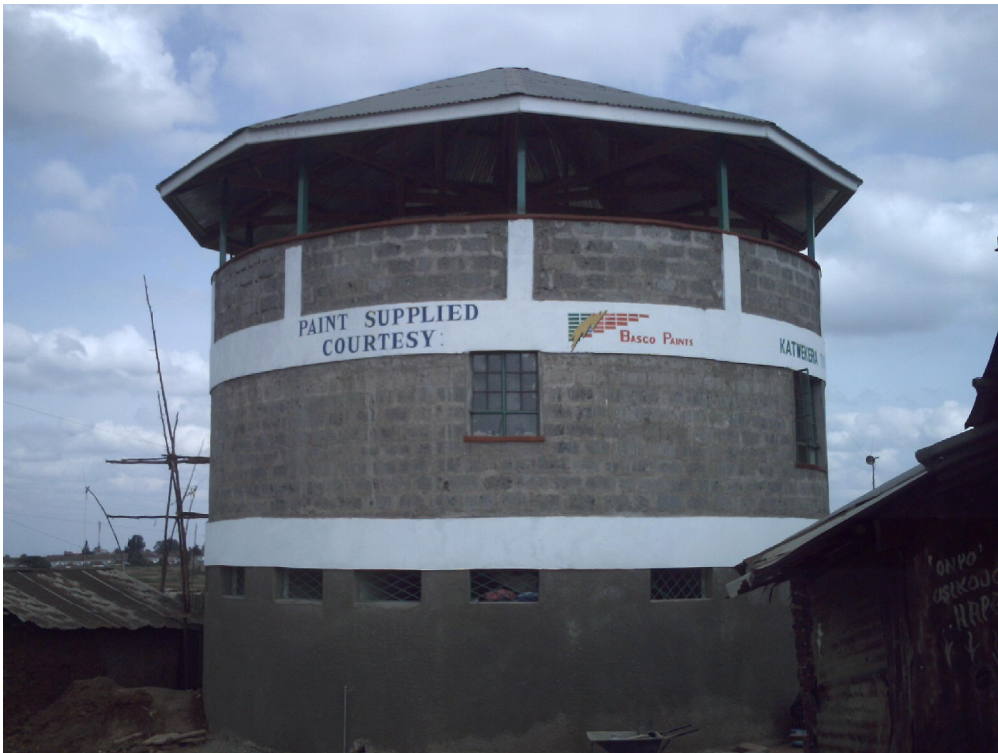
Figure 1. Community-managed sanitation block in Gatwekera village, Kibera, Nairobi. The ground floor is the sanitation compartment, and the top floor is a 'community room' used for meetings, weddings, parties, etc. Underneath the ground floor is ...
