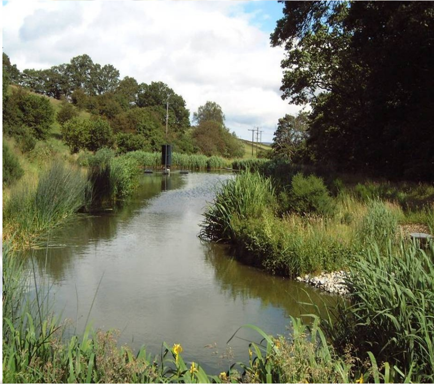
Figure 4.12. Primary facultative pond at Botton Village, near Castleton, North Yorkshire, showing marginal planting.
