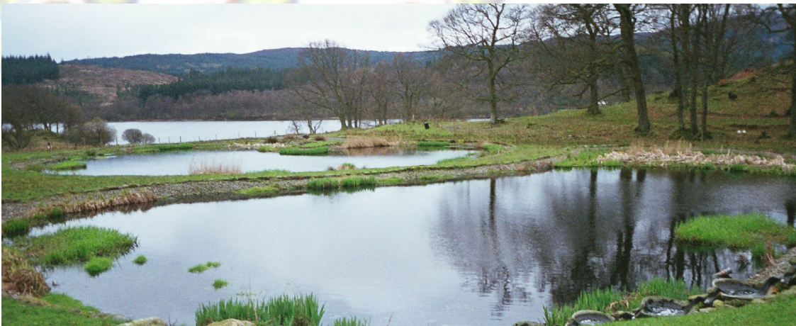
Figure 4.1. The primary facultative pond at Tigh Mor Trossachs, Perthshire, serving a holiday home complex (top). The facultative pond is followed by two maturation ponds (bottom). The final effluent discharges into Loch Achray (beyond the second maturation pond)
