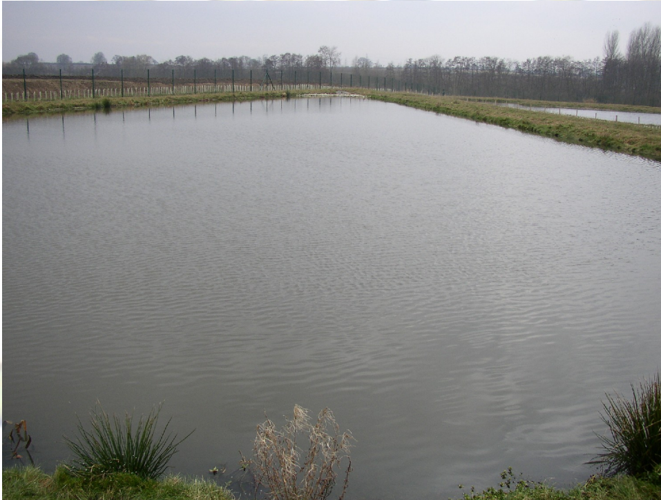
Figure 4.2. Primary facultative pond at Scrayingham, North Yorkshire Pond design by Iris Water and Design, Castleton, North Yorkshire The Scrayingham WSP won Yorkshire Water the 2005 ICE Yorkshire Award and the 2005 BCIA Environmental Award (Kitching, 2005; BCIA, 2005)
