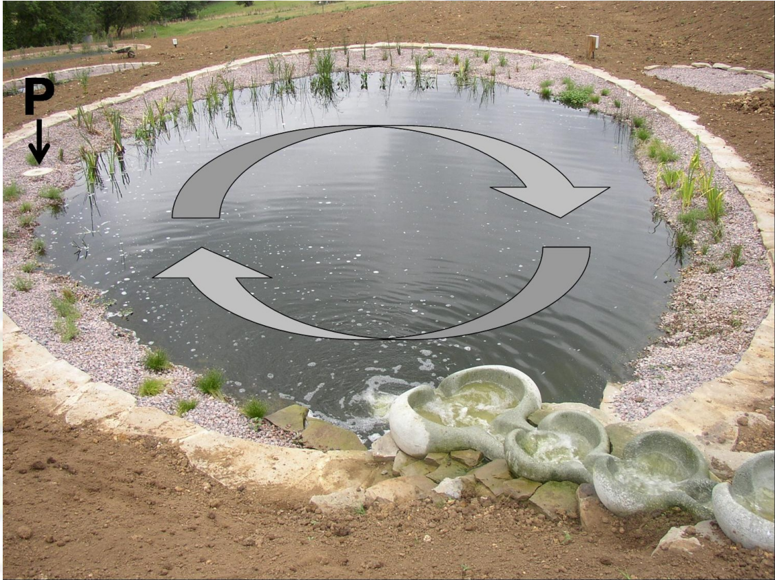
Figure 4.8. One of the four secondary facultative ponds at Hawkwood College, near Stroud (see also Figure 1.2). The pond contents are internally circulated by a 200-W submersible pump (housed at P) which pumps the contents at a rate of ~100 l/min to the top of the ‘flowform’ cascade (bottom left). This induces a gentle circular motion in the pond. (A similar cascade can be seen in the primary facultative pond shown in Figure 4.1.) Each of the four ponds has a different design of cascade, each of which induces a slightly different circulation pattern in the pond; this will permit the ‘best’ system, in terms of performance and biodiversity, to be established. Apart from treating wastewater, the idea of this WSP system was to produce a very aesthetic, tranquil locality for contemplation and meditation (a bench will be located on the small gravelled area shown in the top right corner).
