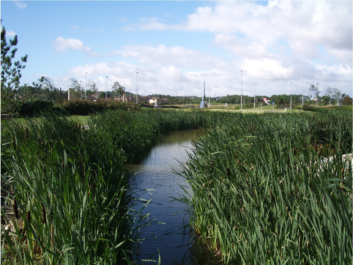
Figure 3.5. Free-water-surface constructed SUDS wetland at Appleton Court, Wakefield, West Yorkshire
