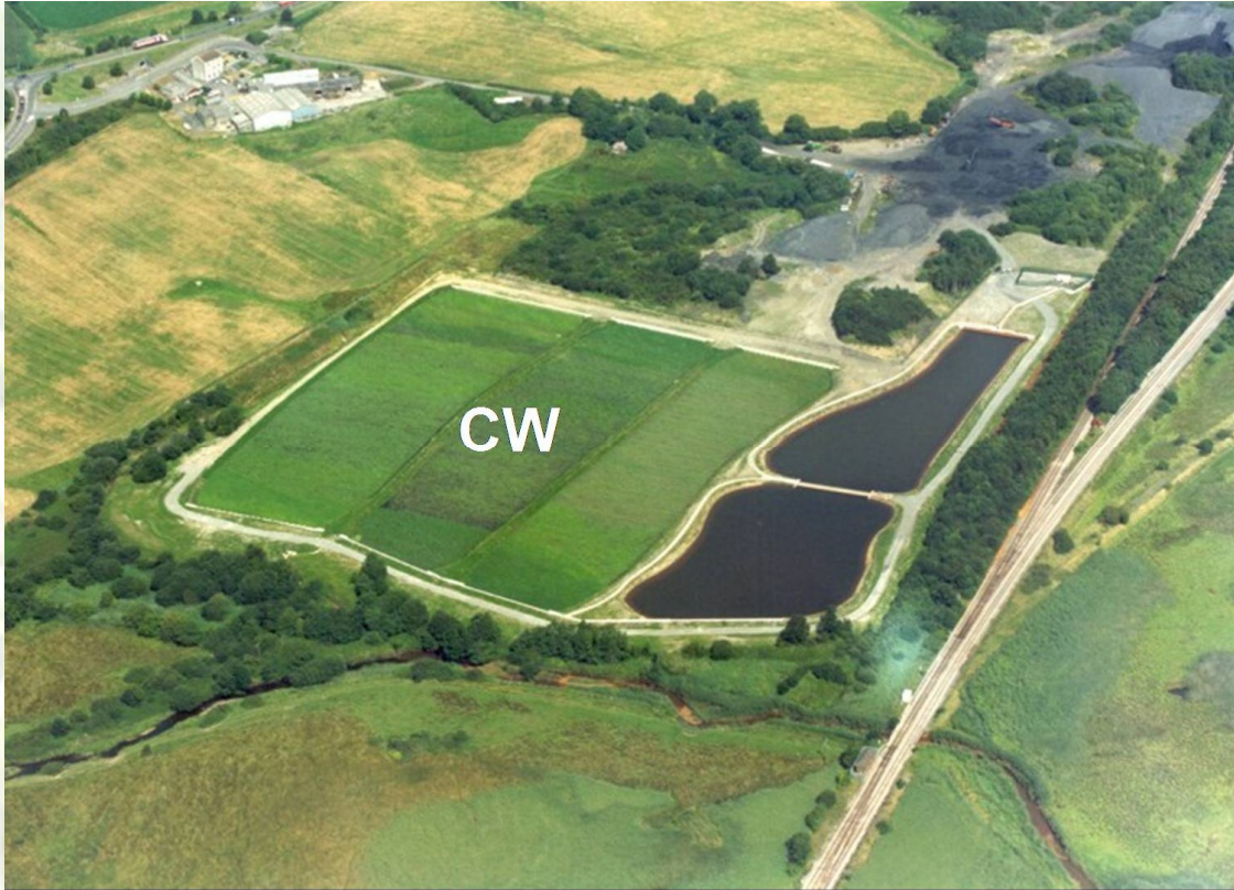
Figure 3.1. Free-water-surface constructed wetlands treating acid mine drainage water at Morlais, Swansea.
