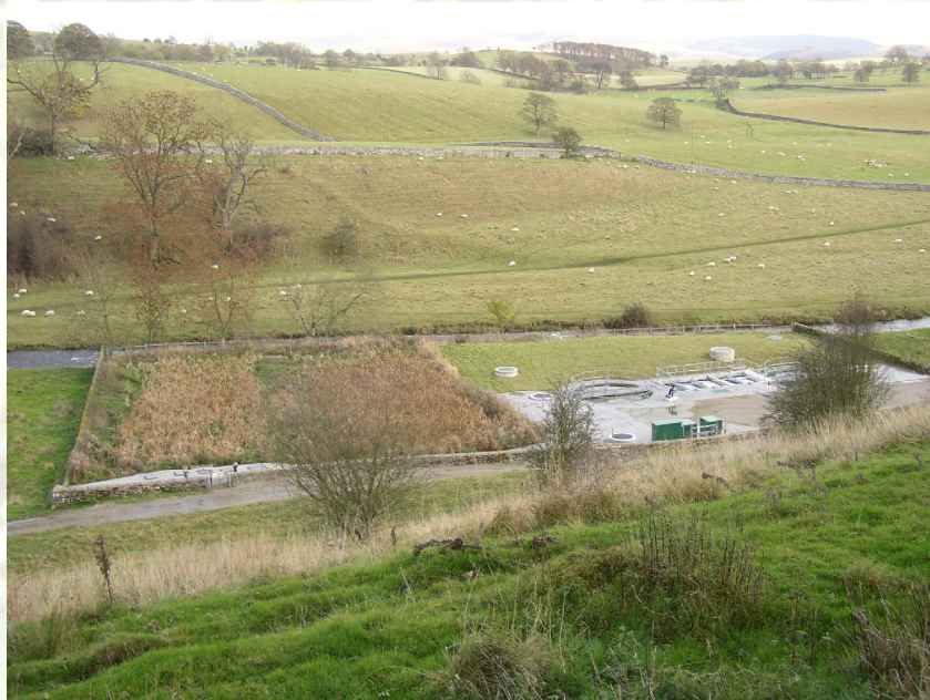
Figure 3.3. Subsurface horizontal-flow constructed wetland at Airton, North Yorkshire in winter (Figure 1.1 shows this CW in summer).
