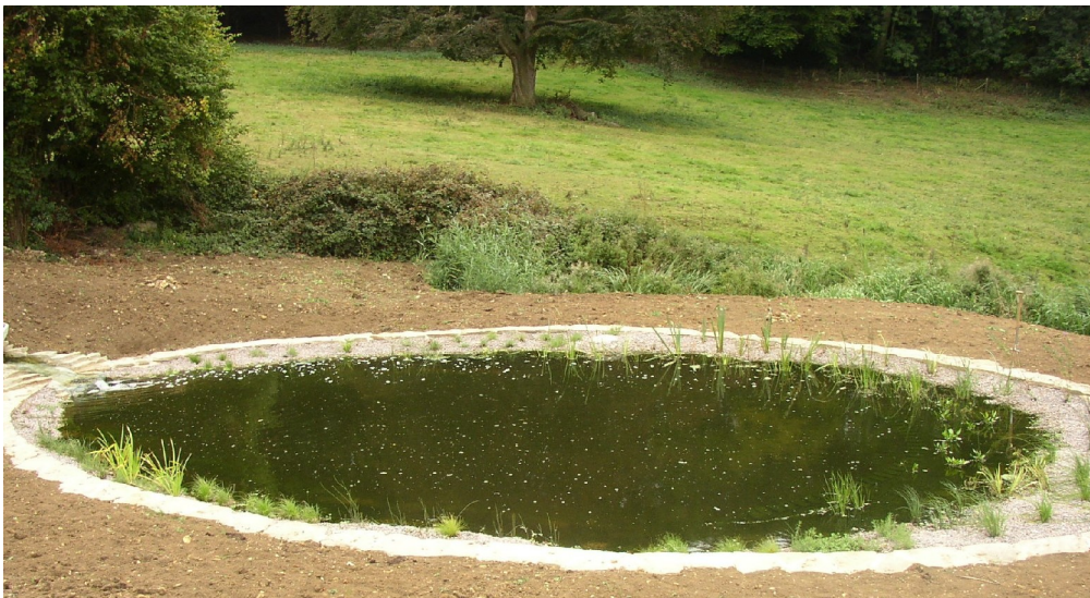
Figure 1.2. One of the four secondary facultative ponds at Hawkwood College, near Stroud, shortly after commissioning and planting of the marginal plants in August 2005 (see also Figure 4.8). Pond design by Ebb & Flow Ltd, Nailsworth, Gloucestershire.
