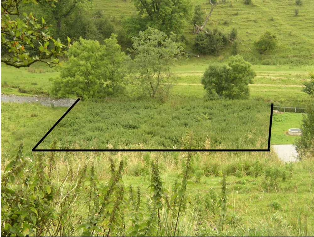
Figure 1.1. Constructed wetland (within the black lines) at Airton wastewater treatment works, North Yorkshire
