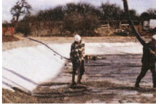
Figure 7.3 Facultative pond embankment
