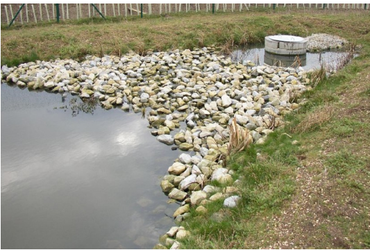
Figure 6.3 Facultative pond rock filter
