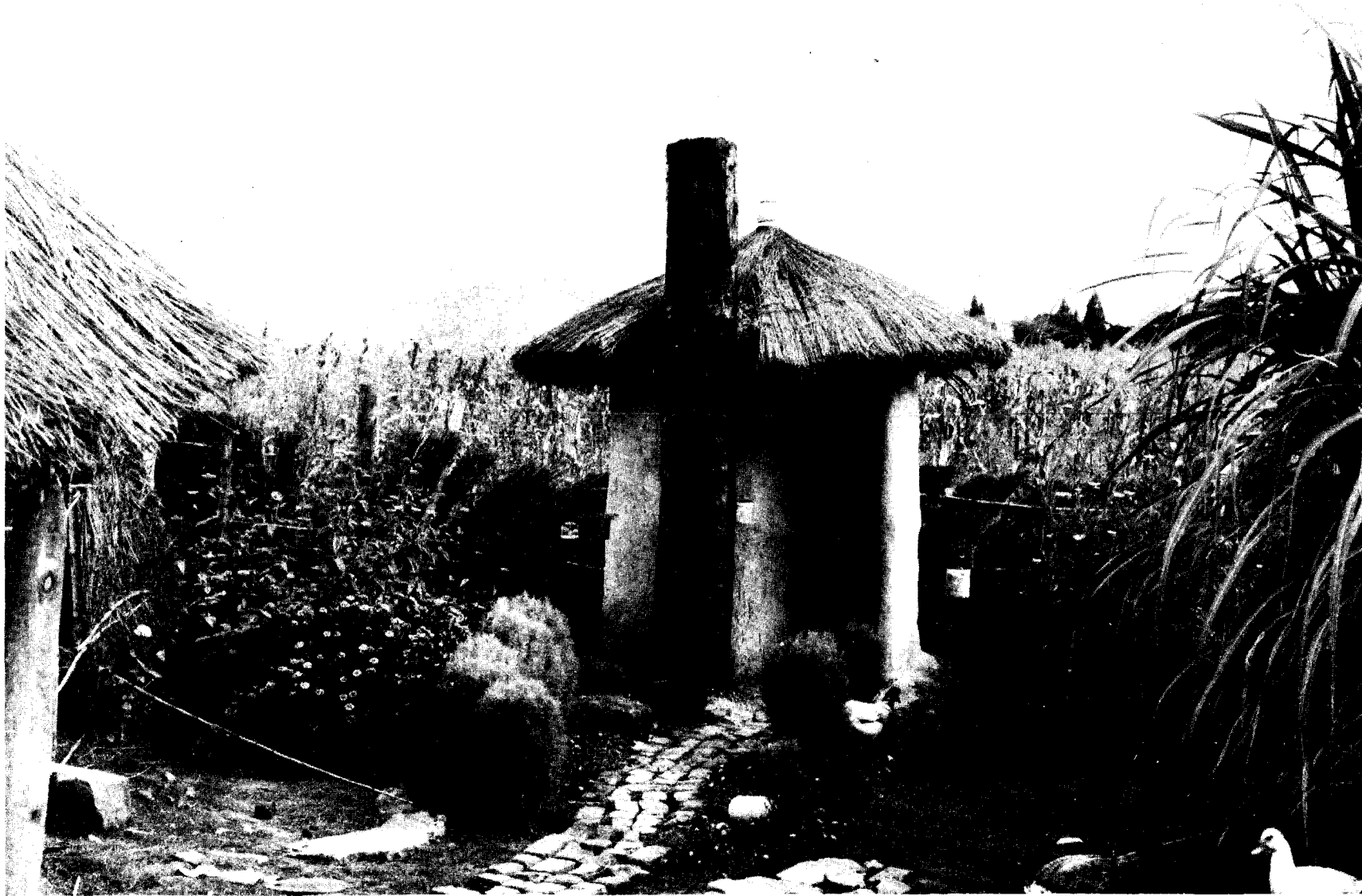
Figure 10: Mud and wattle spiral VIP latrine.
