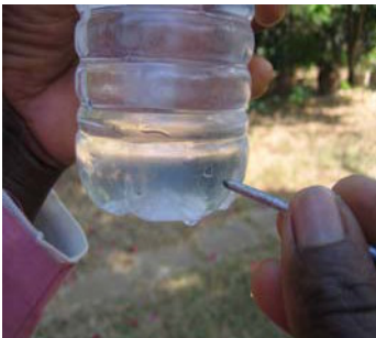
Figure 9-8: Piercing a hole in the plastic bottle
