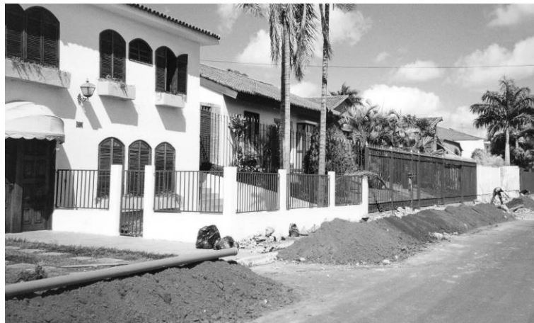
Figure 1: Simplified sewerage being installed at the back of the pavement in Brasilia
