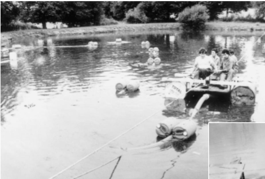
Figure 8.2 Pond desludging in northern France using a raft-mounted sludge pump. Detail: sludge suction head
