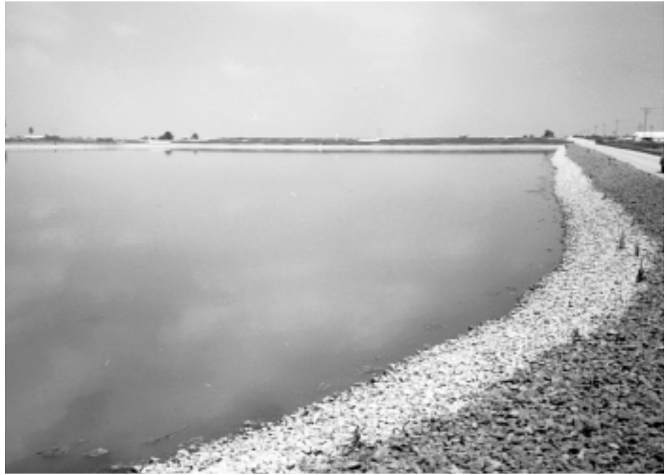
Figure 7.2 Embankment protection by stone rip-rap
