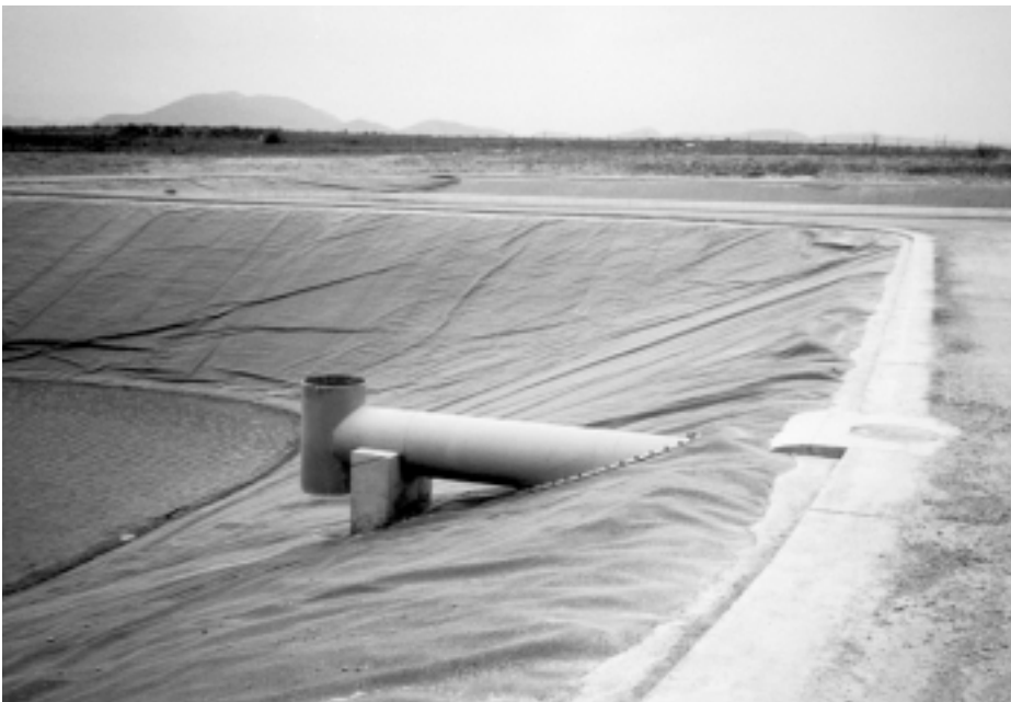
Figure 7.3 Anaerobic pond lined with an impermeable plastic membrane
