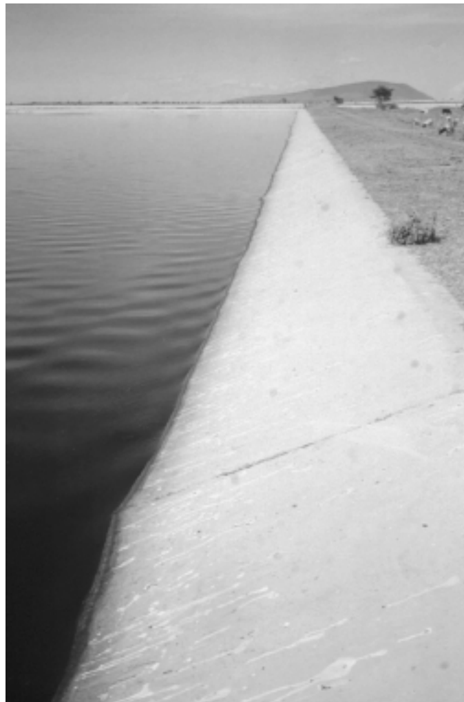
Figure 7.1 Embankment protection by in situ -cast concrete
