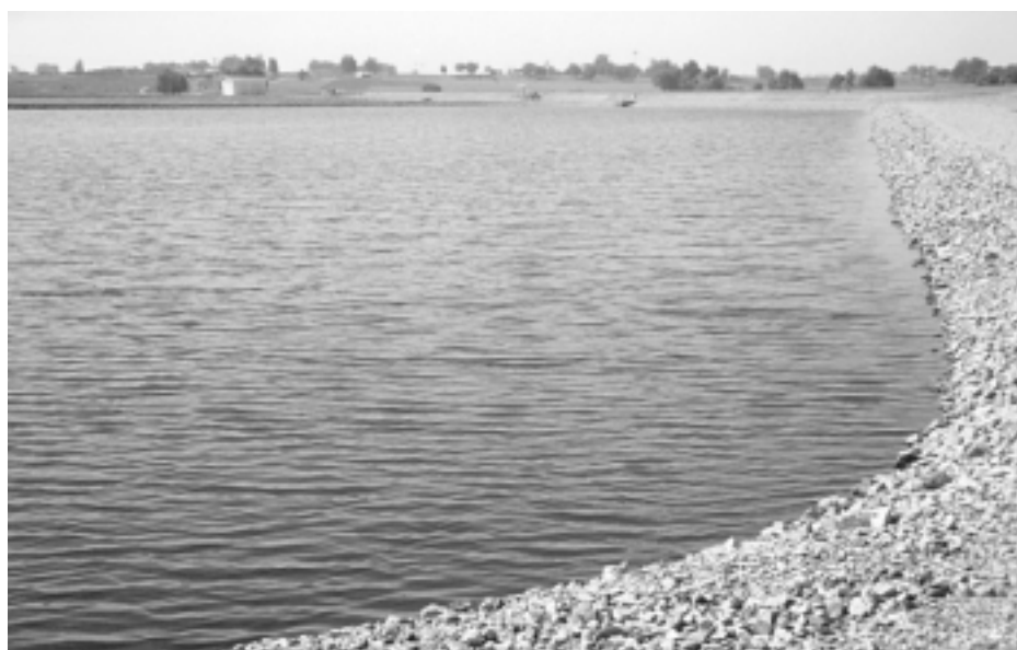
Figure 5.7 Storage reservoirs at Ben Slimane
