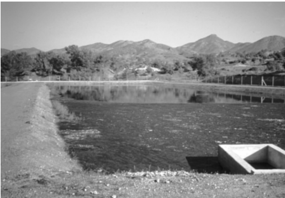
Figure 4.3 Anaerobic pond at Kophinou treating slaughterhouse wastewater
