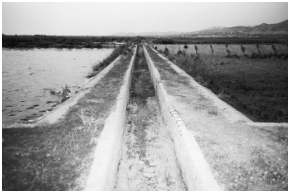
Figure 4.1 Primary facultative ponds at Sereflikochisar - that on the right has been emptied and desludged. The central channel is a flow by-pass facility
