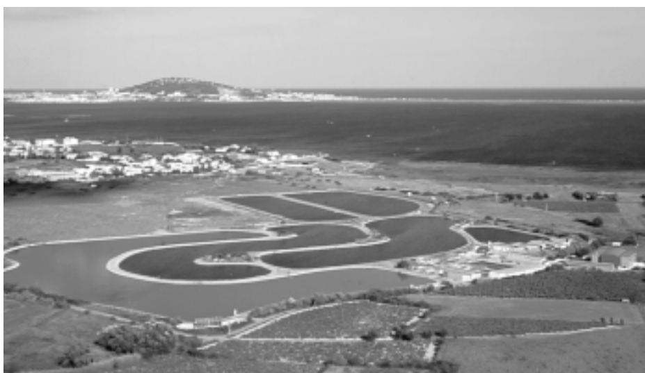
Figure 3.3 The WSP at Mèze, near Montpellier
