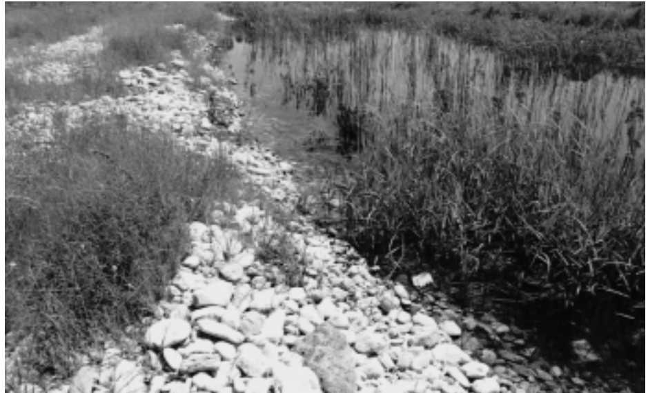
Figure 3.5 Rock filter in the secondary maturation pond at Kokinixoma
