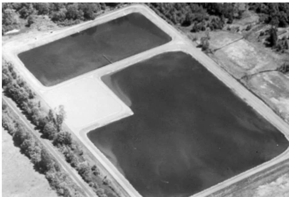
Figure 10.2 Rock filter installed in the corner of a pond at Veneta, Oregon, USA
