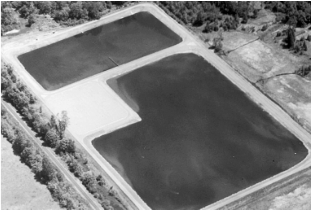
Figure 8.2 Rock filter installed in the corner of a pond at Veneta, Oregon, USA.
