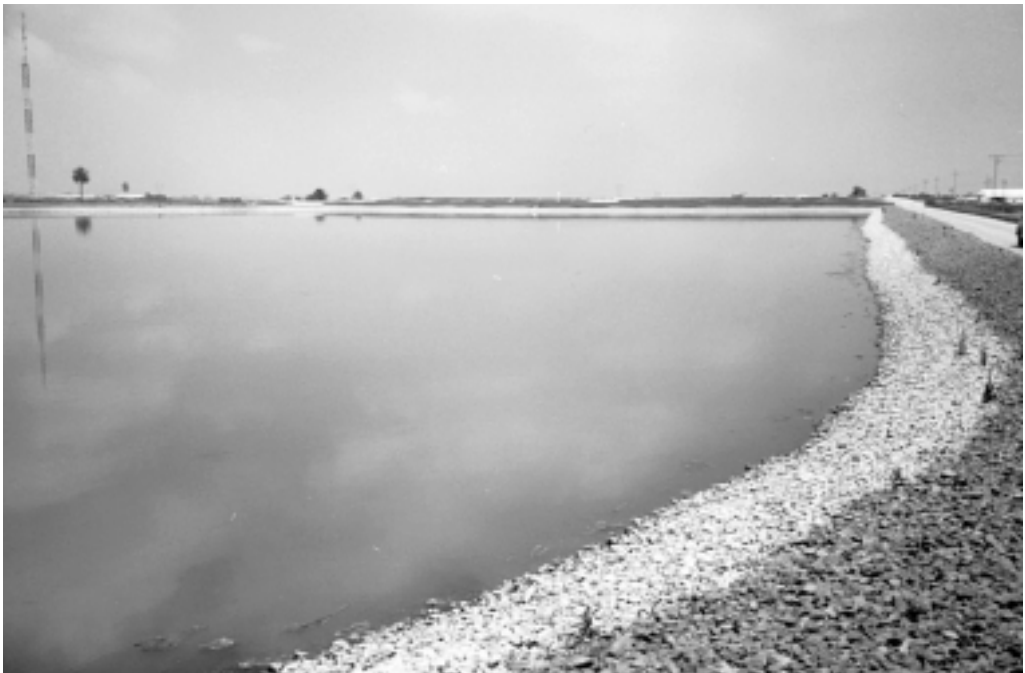
Figure 5.2 Embankment protection by stone rip-rap.
