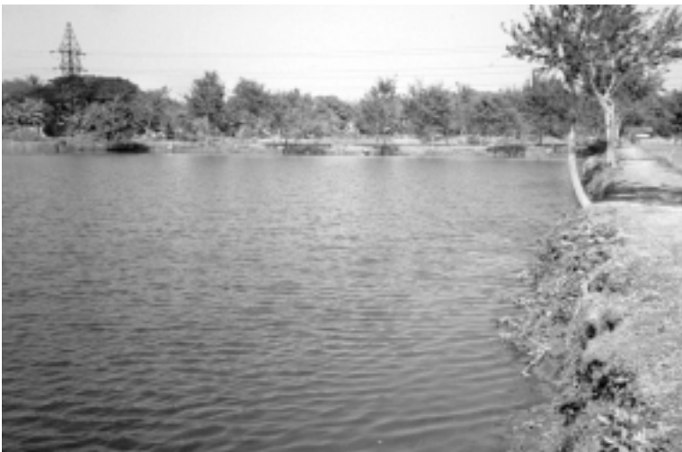
Figure 2.1 View of WSP at Titagarh in the metropolitan Calcutta area.
