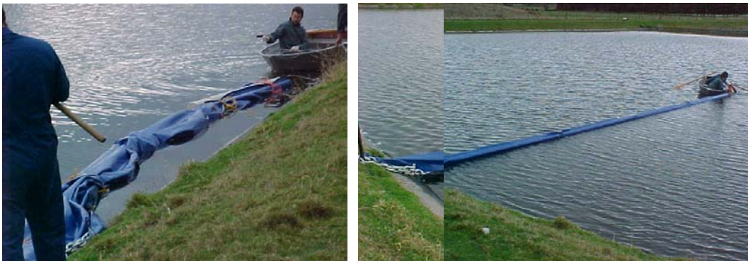
Figure 9-4 Baffle being installed at Ashhurst secondary pond
