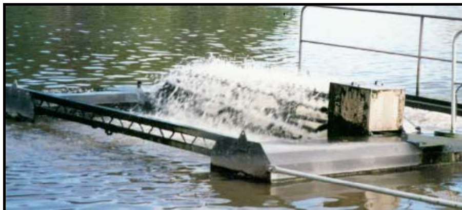
Figure 7-2 Example of an aerator
