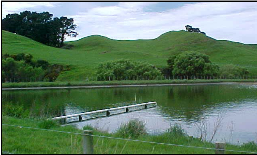
Figure 4-6 Field pond with inflow dropping from a horizontal pipe
