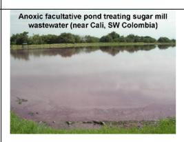
Facultative ponds, like this one in southwest Colombia, turn purple when they are overloaded. So much sulphide is produced that the algae are inhibited (in fact, by the high level of dissolved H<sub>2</sub>S gas), and concomitantly there is a huge growth of photosynthetic bacteria as they quickly respond to the greatly increased concentrations of sulphide, so the pond turns purple.
