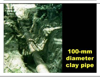
100-mm diameter clay pipes were used, simply because at that time in Natal these were cheaper than PVC pipes.
