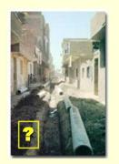
It is very important to use the correct sewer diameter because **small wastewater flows flow better in small sewers.** However, national sewerage design codes often specify a larger-than-necessary sewer diameter, but in fact we know from over 25 years' experience in northeast Brazil and elsewhere that 100 mm sewer diameter *is* OK, and this is the minimum that we normally use.
