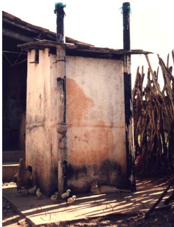
Plate 4.67. A septic tank/bathroom unit
