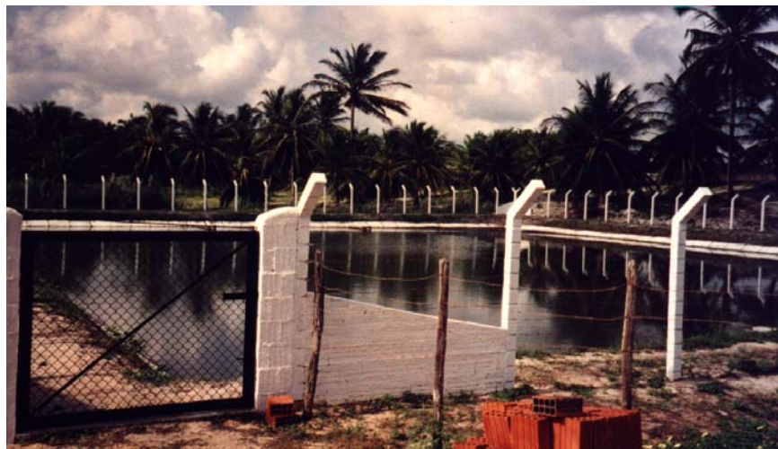
Plate 4.74. Waste stabilisation pond at Juritianha
