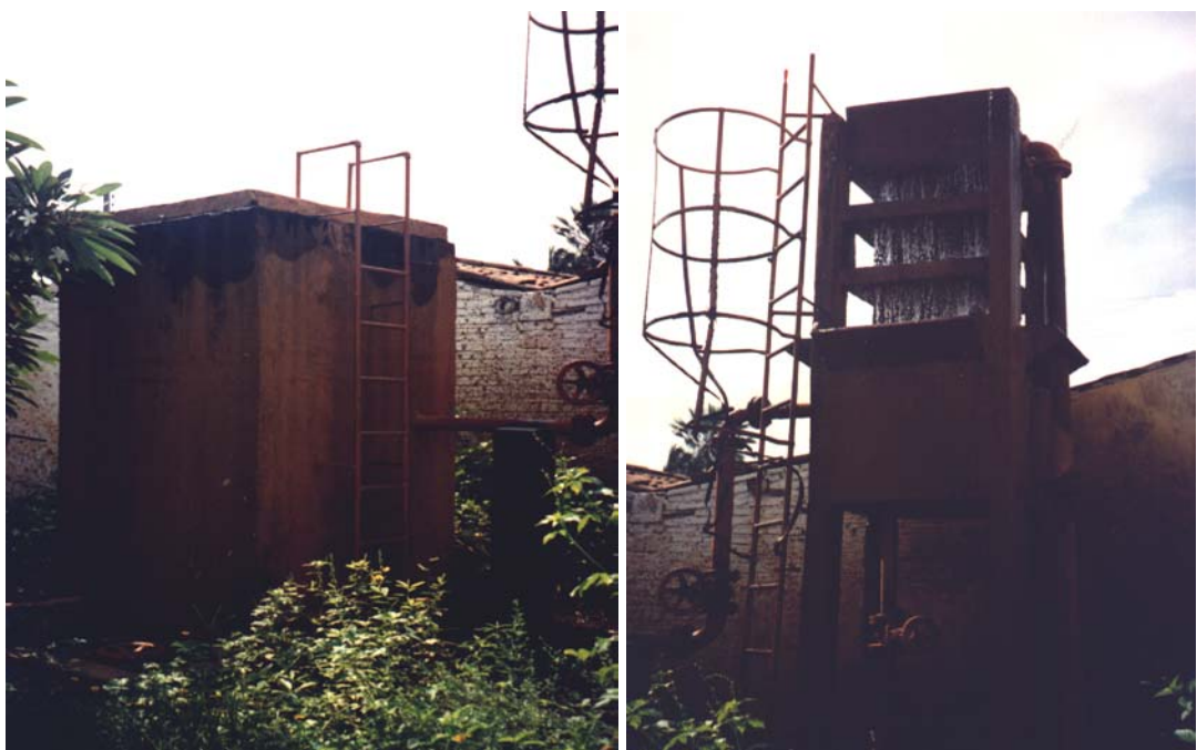
Plate 4.72. The aeration and sand filtration of the water treatment plant at Parapui
