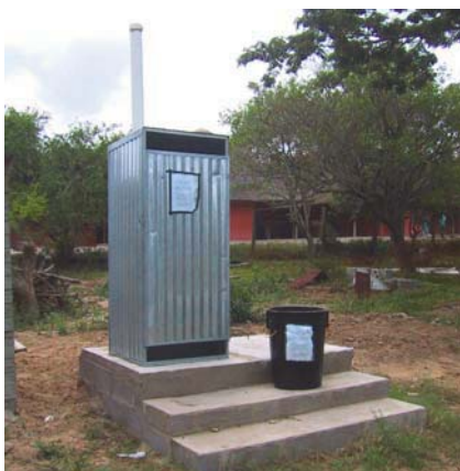
Figure 4-27: Fossa alterna with a metal structure
