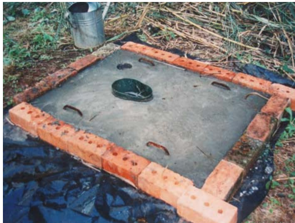
Figure 4-7: The completed slab inside the mould
