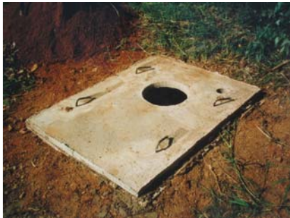
Figure 4-13: Addition of the concrete slab
