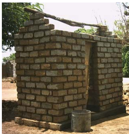
Figure 4-28: Brick double pit composting toilet
