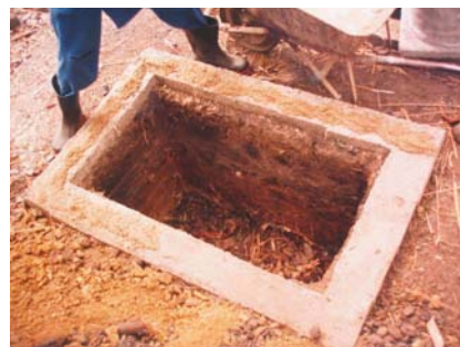
Figure 4-12: Completed Fossa alterna pit
