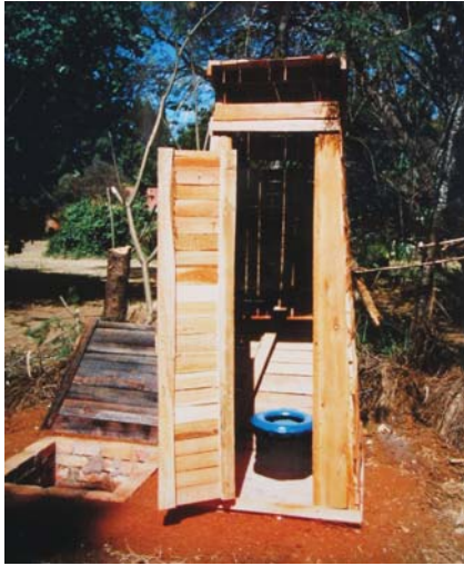
Figure 4-15: Fossa alterna using a wooden structure
