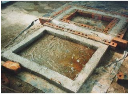
Figure 4-9: Ring beam mould using bricks
