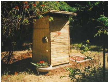
Figure 4-1: A portable structure using poles and reeds
