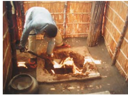
Figure 4-22: Excavating the humus from the pit
