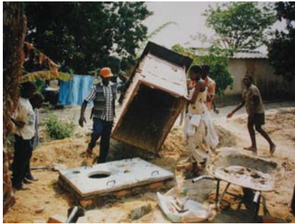
Figure 4-19: Fitting a portable superstructure to a Fossa alterna pit
