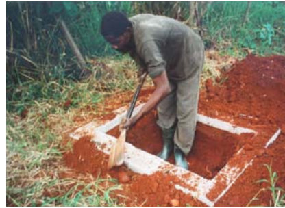
Figure 4-10: Digging the pit for the Fossa alterna
