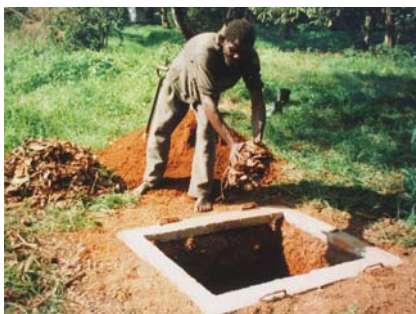
Figure 4-11: Adding leaves to the Fossa alterna pit
