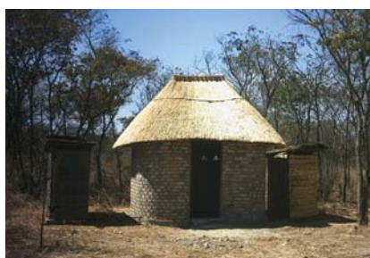
Figure 4-26: A Fossa alterna with a permanent brick and thatch structure
