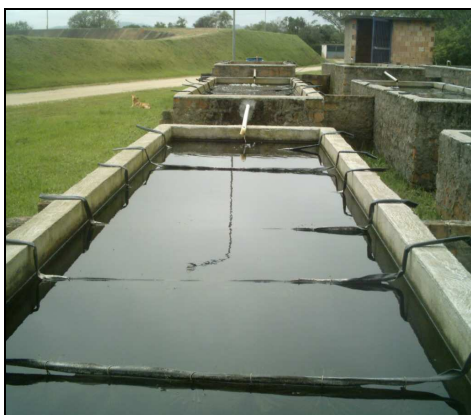
Figure 01- View of an individual module and support brushes
