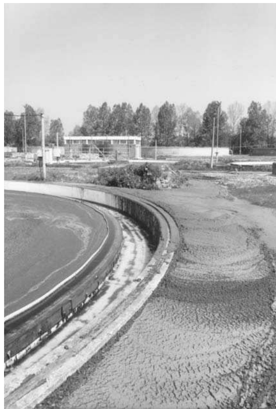
Fig. 32.4 A Microthrix parvicella foam illustrating the risk placed upon effluent quality and safety.
